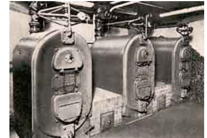
A boiler house from 1932.
