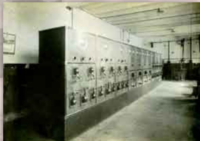
The main switch panel on-board the 'Sibagak' in 1927.
