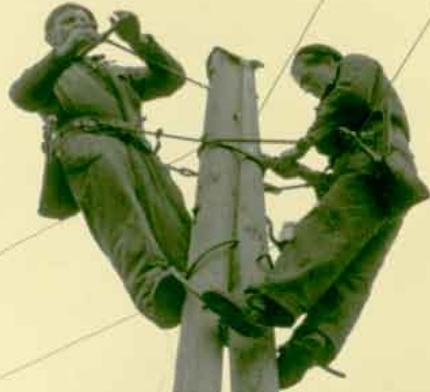
Two Linemen wearing genuine 'climbing skates' working on the above ground electricity network in the 1930s.
