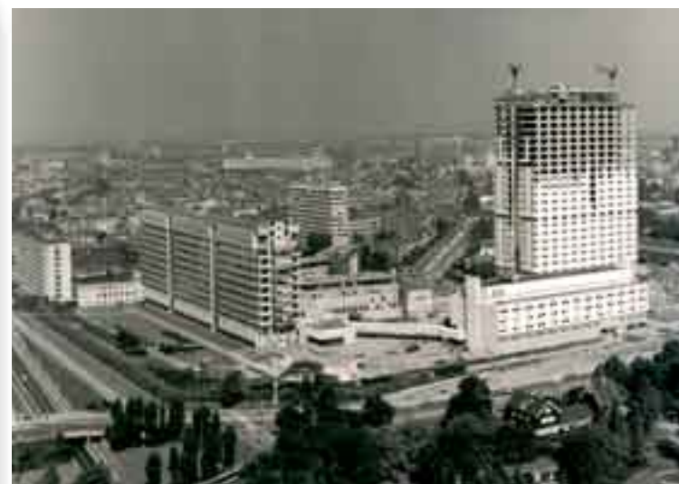
The new Erasmus Ziekenhuis (hospital) in Rotterdam was built in 1968. Van Rietschoten & Houwens supplied all the electrical engineering solutions.
