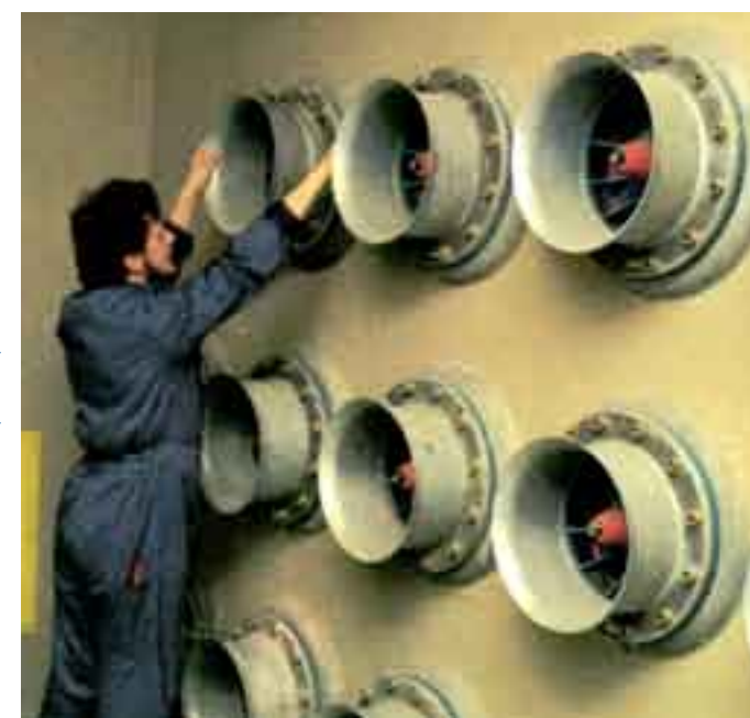
Lier Town Hall was an important reference for ABI. The climate control systems had anti-nuclear explosion valves and the cellar could serve as an atom bomb shelter.
