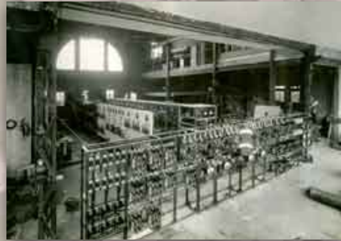
Van Rietschoten & Houwens' workshop in 1923 showing the technology for three ships: 'Damsterdijk' (front), the 'Kota Pinang' (centre) and 'Baloera' (rear).
