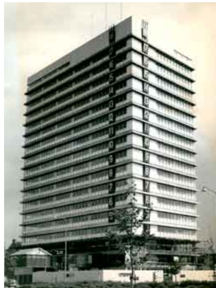
The Ministerie voor Maatschappelijk Werk (Ministry of Welfare) in Rijswijk was built in 1965 using the famous 'Jack Block' building system. In this ingenious logistics process the top floor was built first and the building was then jacked up floor by floor. R&H delivered all electrical solutions.
