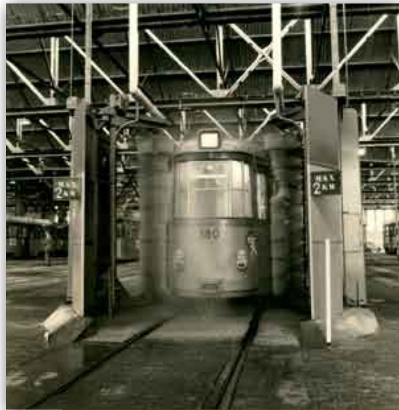
The first automatic tram 'washing machine' in the Netherlands (around 1960).
