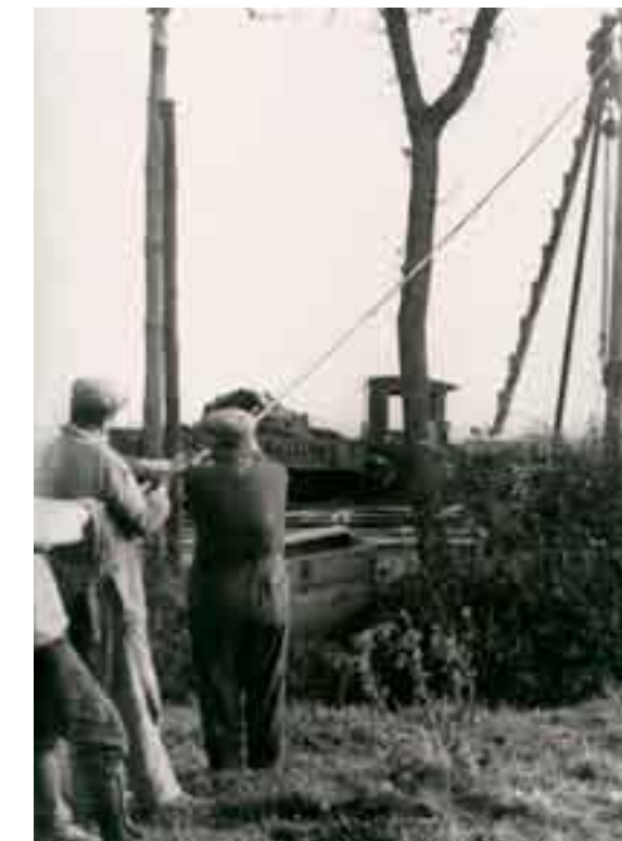
Installing electricity pylons was a specialized profession.
