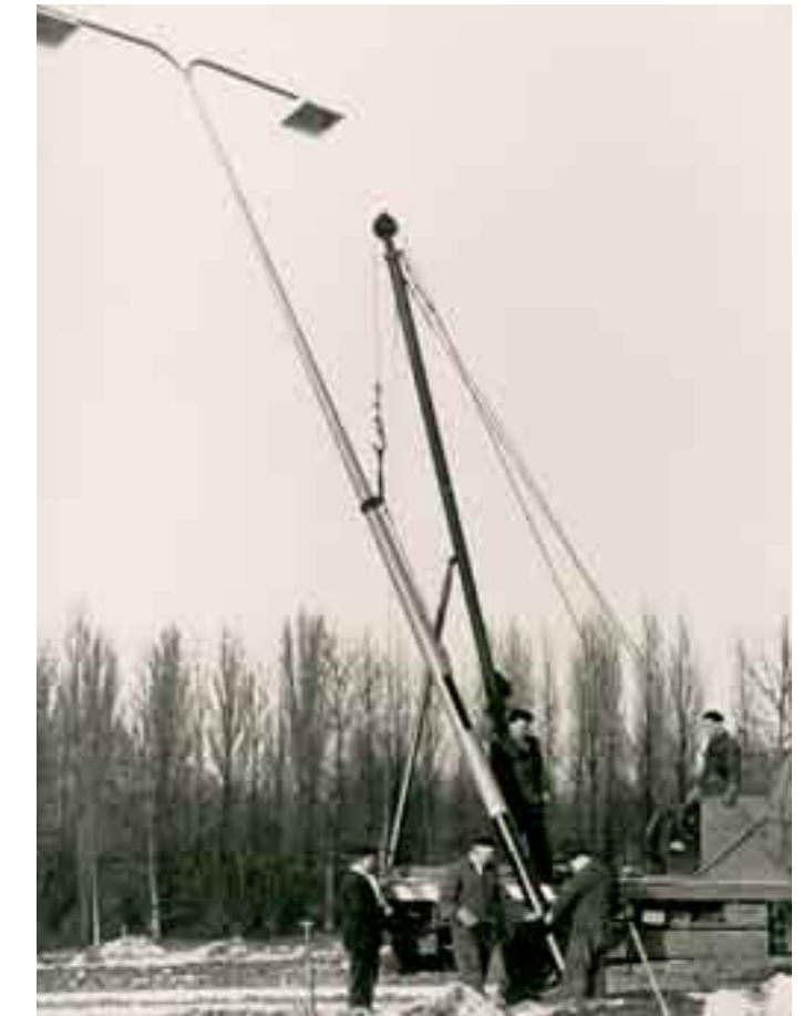
Installing public lighting in the early 1960s.
