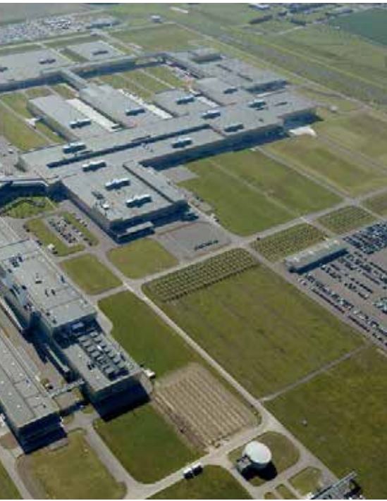
The BMW works in Leipzig is currently undergoing extensions the form of a press shop and a production hall for bodies-in-white. In addition to the 3-series sedans and three 1-series models, the future, all-new X1 will be made in Saxony.
