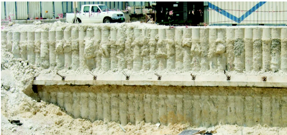
Excavation in Doha with anchored pile wall
