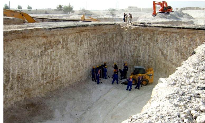
Excavation on a main road to the north
