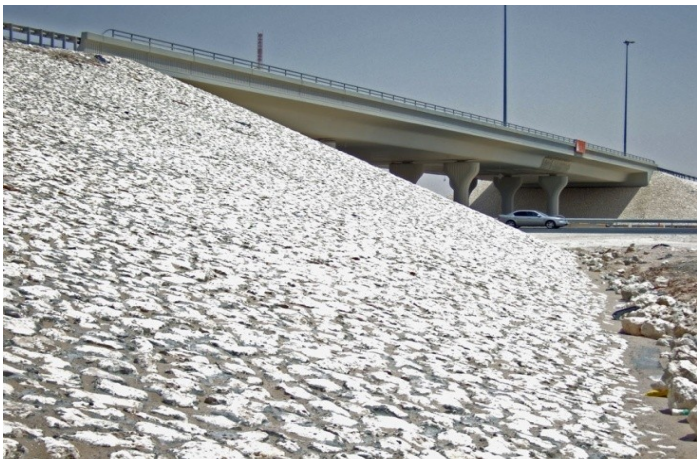
Surface (dam with limestone and mortar bed) Salwa Road
