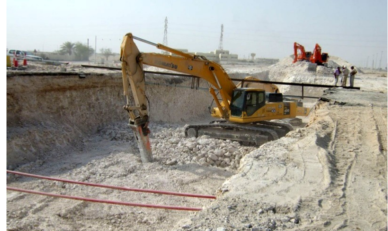
Loosening limestone by chiselling
