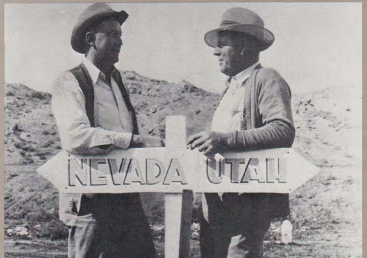
A handshake marks the site of the last link of buried cable spanning the nation in 1943. It was close to the site of the 1914 pole-line linkup.
