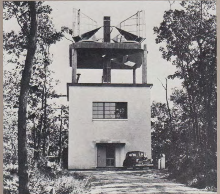
One of the very first microwave radio repeater stations on the route between New York and Boston. This photo is dated November 13, 1947. Very quickly microwave became the backbone of the long distance telecommunications network.
