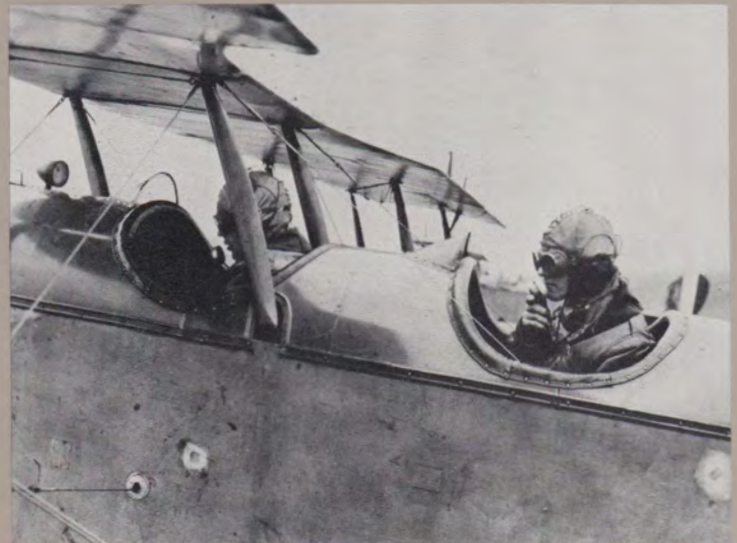
Early air-ground radio experiments conducted by Western Electric during World War I. Prior to the invention of the microphone, a passenger needed strong lungs to communicate with the pilot. Those are fabric patches, not bullet holes that are visible on the fuselage.
