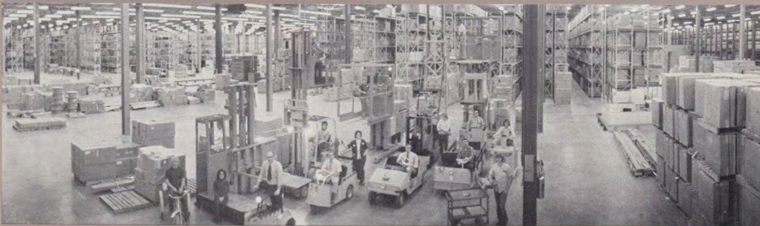
Be w—Seven superwarehouses—one in each Service Region—were built to stock service centers, distribution centers and installation jobs. This one is located in Martinsville, W. Va.
