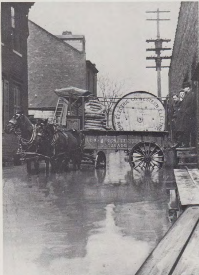
The year was 1913, and a lot of Pennsylvania was under water. This WE cable being loaded in Pittsburgh helped restore communications. So did the two-horsepower wagon.
