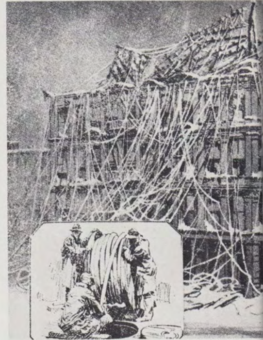
The year we joined the Bell System got off to a frigid and calamitous start with the Blizzard of 1881. The spaghetti swallowing the Boston central office above had to be reconverted into working telephone lines. The inset shows underground cables which "have no fear of ice."
