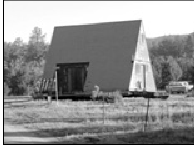
An A-frame on Main Street, on its way to another part of Timberon.
