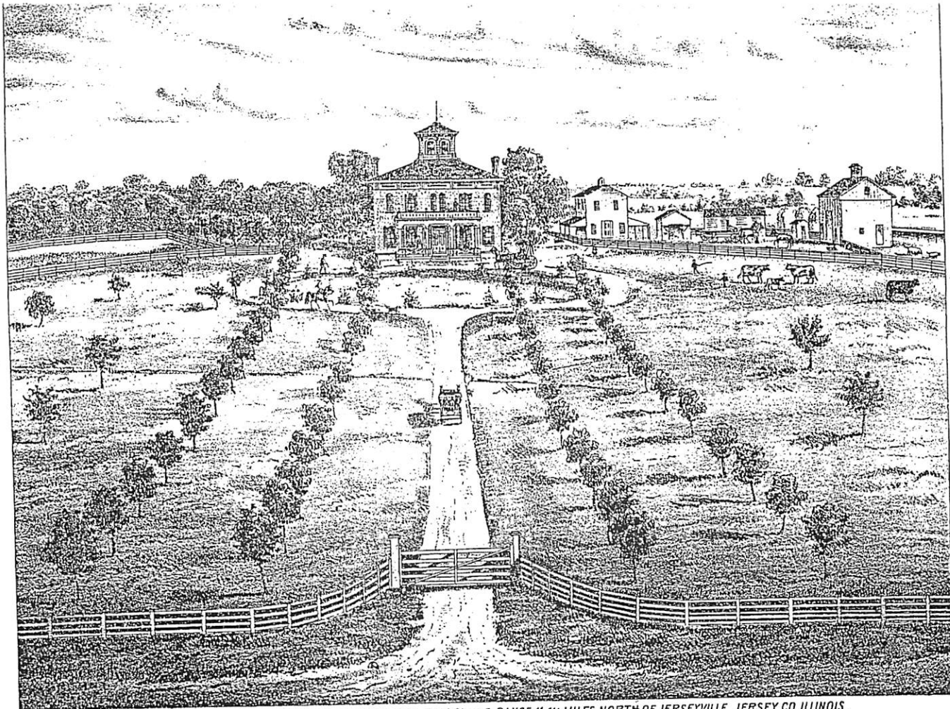
COUNTRY RESIDENCE OF C.B. FISHER SECTION 17 TOWNSHIP 8 RANGE 11 1/2 MILES NORTH OF JERSEYVILLE JERSEY CO. ILLINOIS.
