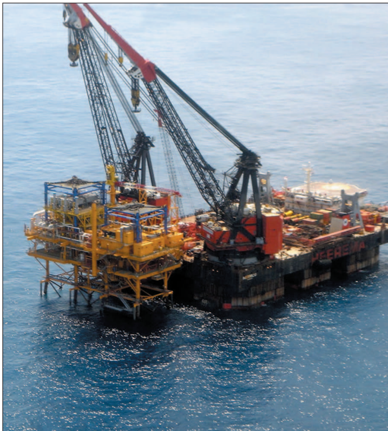
The giant semisubmersible crane vessels – Balder (left) and Hermod (right) – in their North Sea prime. Balder is pictured installing two modules simultaneously on the Ninian Northern platform, 1979.
