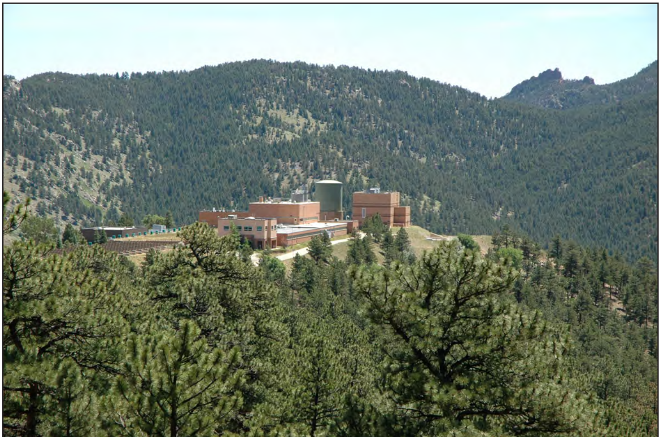
The Betasso Water Treatment Plant. Pettem photo, 2013
