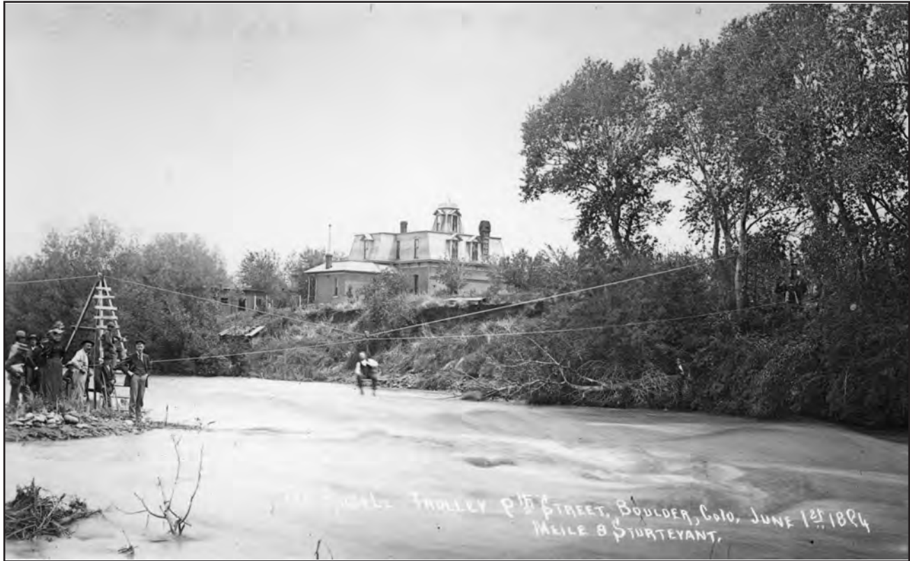
After all of the bridges had washed out in the 1894 flood, this makeshift conveyance transferred people (and kegs of beer) across Boulder Creek. Carnegie Branch Library for Local History, Boulder Historical Society collection (225-1-8)
