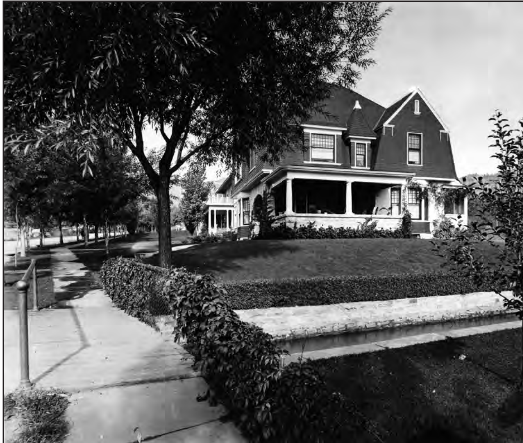
Farmers Ditch (visible in the foreground) was built in 1862, and its water was piped into Boulder homes beginning in 1872. This photo of 637 Pine Street was taken in 1973. Carnegie Branch Library for Local History, Boulder Historical Society collection (207-14-7#1)
