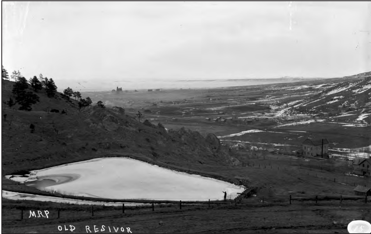
Above, the Town of Boulder Reservoir, built in 1875, was also known as the Red Rocks Reservoir and Sunshine Reservoir #1. The use of the name "Sunshine" is misleading, as the site is accessed through today's Settlers' Park, off of Pearl Street. The Yount flour mill is in the right center of the photo. Carnegie Branch Library for Local History, Boulder Historical Society collection ( S-936)
