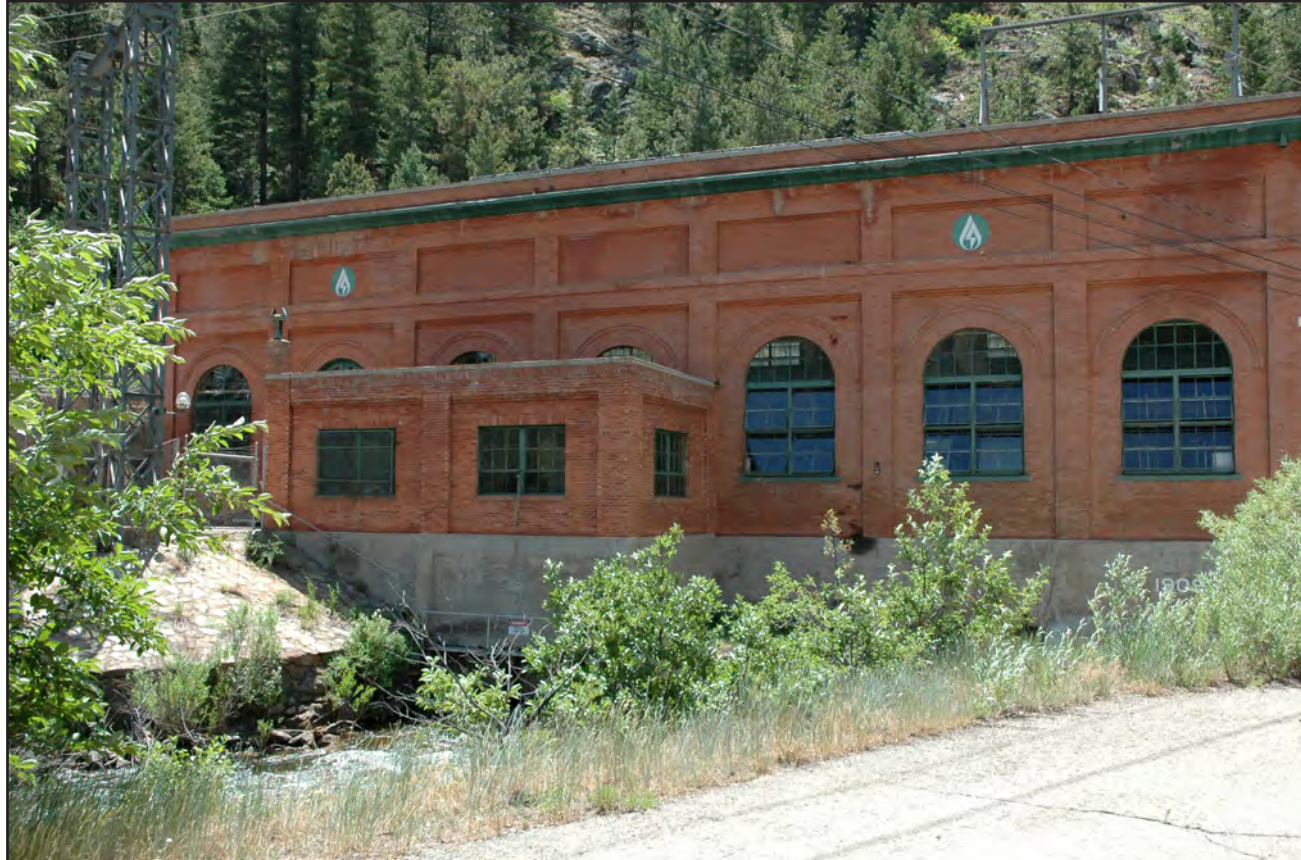
The exterior of the Boulder Canyon Hydro Plant has changed very little since 1910. Pettem photo, 2013
