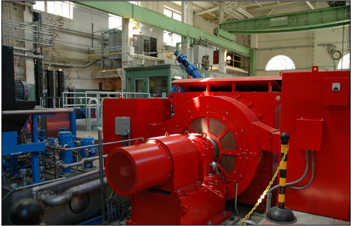
Above, a new generator and turbine, installed in the Boulder Hydro Plant, in 2012, replaced “Unit B”—one of two units dating from 1936. While keeping up with the latest technologies, the future of Boulder’s waterworks also builds on its past. The photo, below, of the Boulder Canyon Hydro Plant was taken in 2013. Pettem photos , 2013
