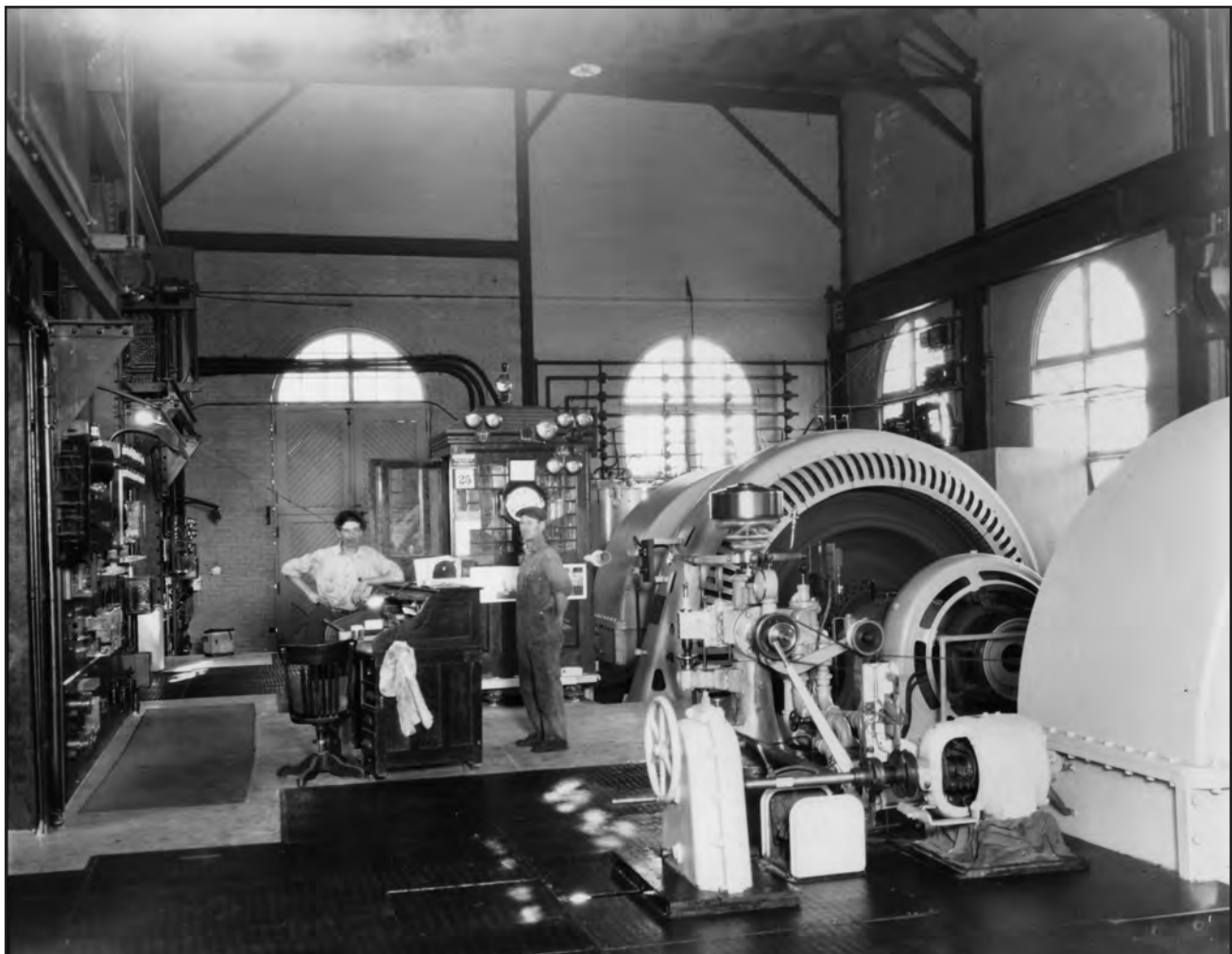
One of the two original generators was photographed in 1924. The generators, installed in 1910, were replaced in 1936 (see following page). Carnegie Branch Library for Local History, Boulder Historical Society collection (141-2-9)
