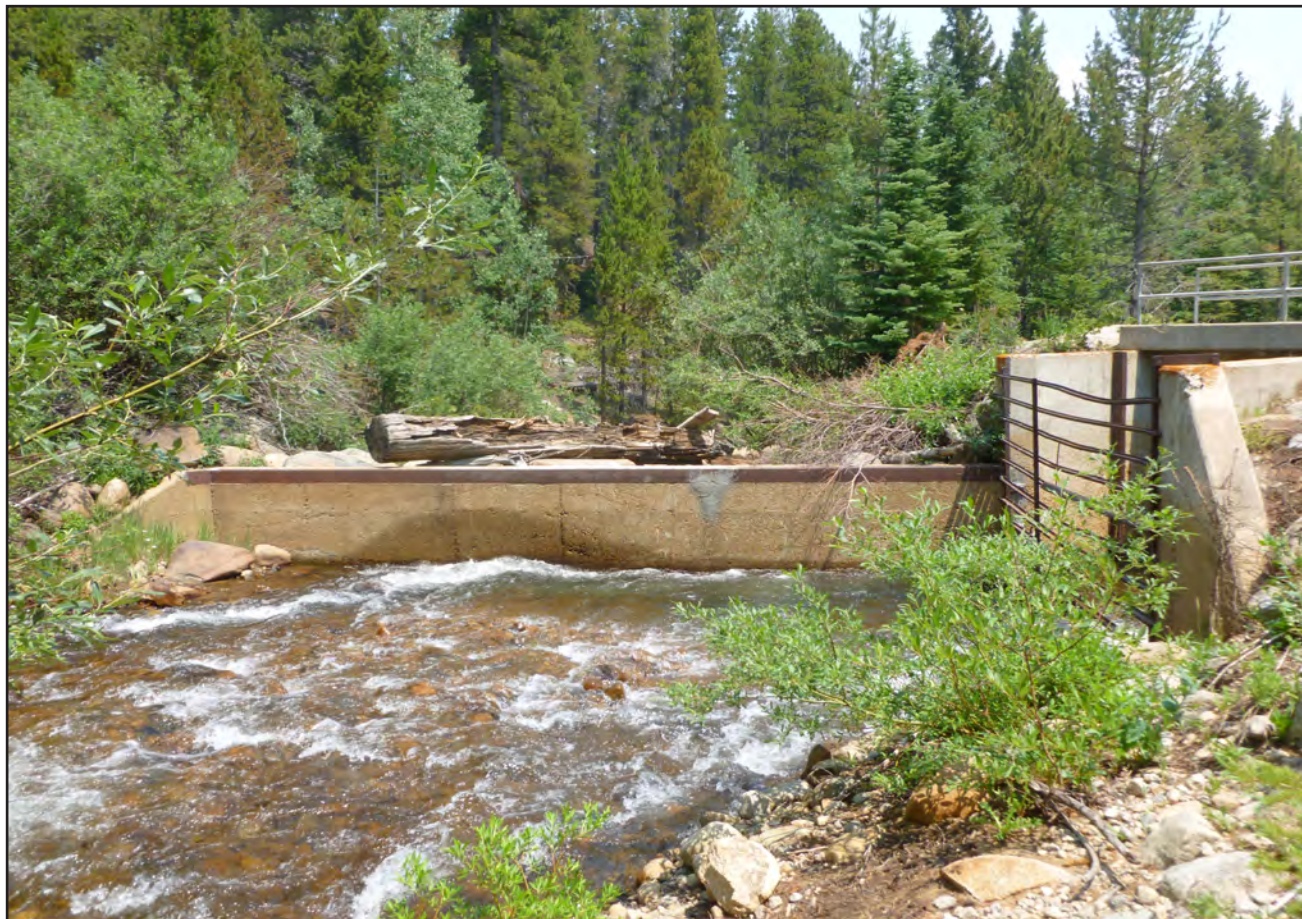
This 2012 photo, or the headgate of Left Hand Ditch, shows the diversion dam that moves water from the South St. Vrain Creek into the Left Hand Ditch. Courtesy Donlyn Arbuthnot
