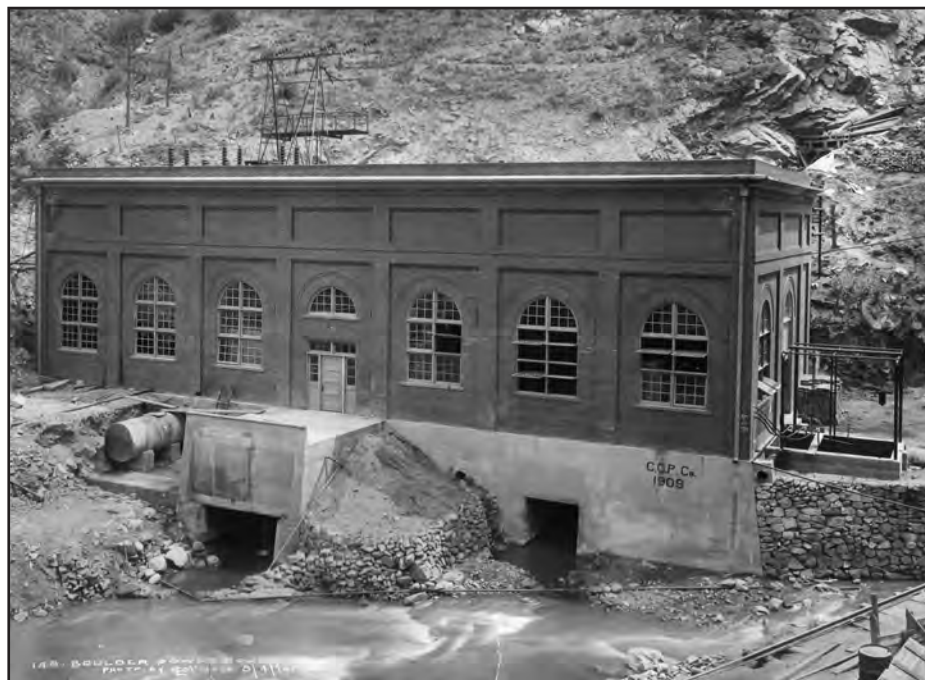
Luckily, L.C. McClure, a well-known photographer, was on hand on August 4, 1910 for opening day at the Boulder Hydro Plant. Photos courtesy City of Boulder.
