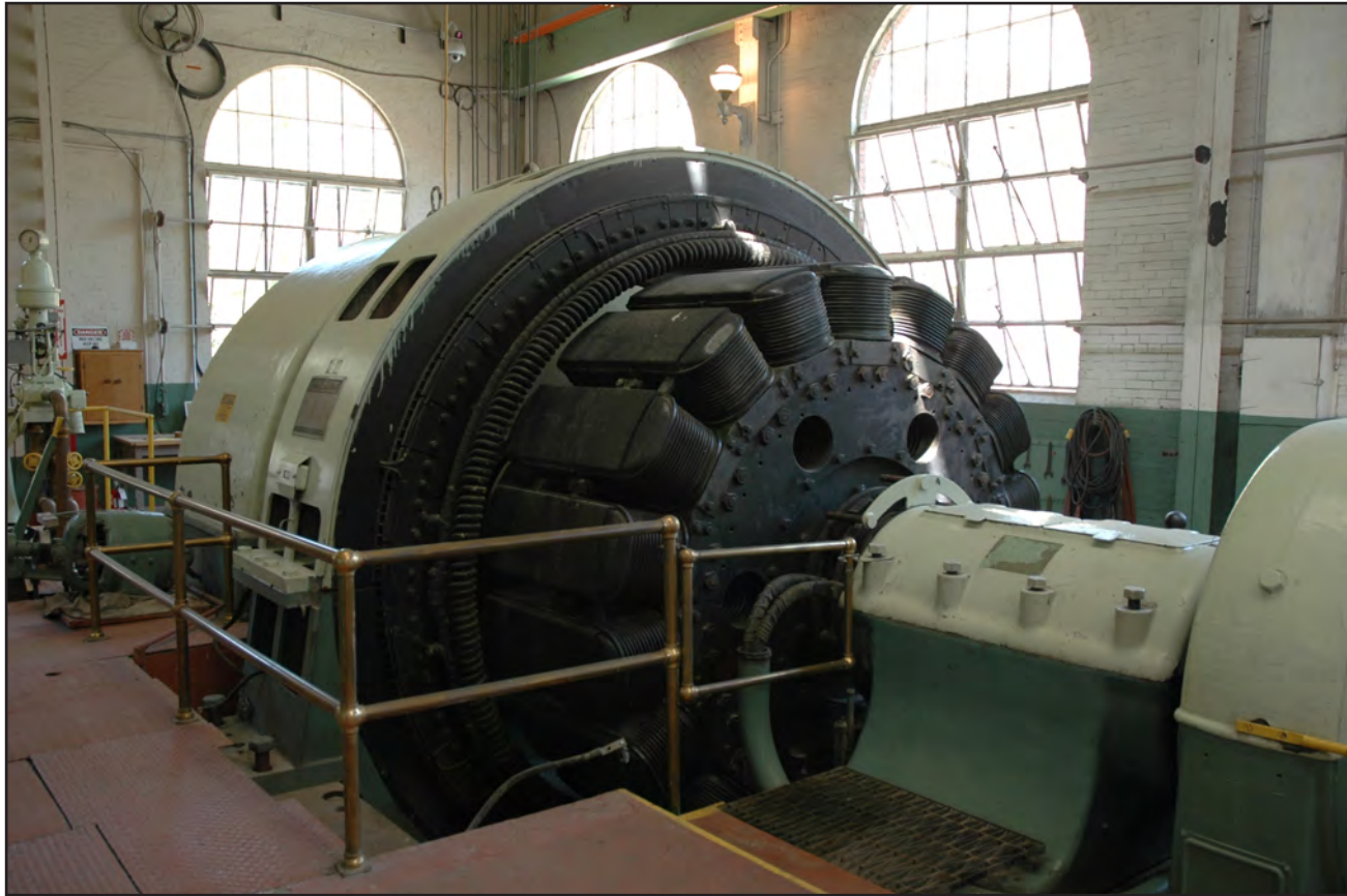
Above, two 400 rpm GE 10 Mw synchronous generators were installed in 1936 to replace the original units (see preceding page). This generator ("Unit A") is no longer functional, but it remains in the Boulder Canyon Hydro Plant for historic preservation. (The other unit was replaced in 2012.) Below, the overhead crane dates from 1910. Pettem photos, 2013
