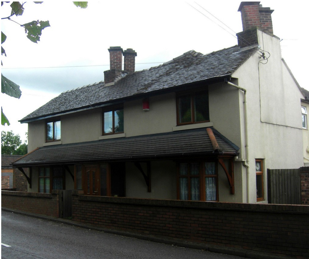
SJ 753 474. Lower Winehill Tollhouse on A531. Nantwich to Newcastle-under-Lyme Trust.
