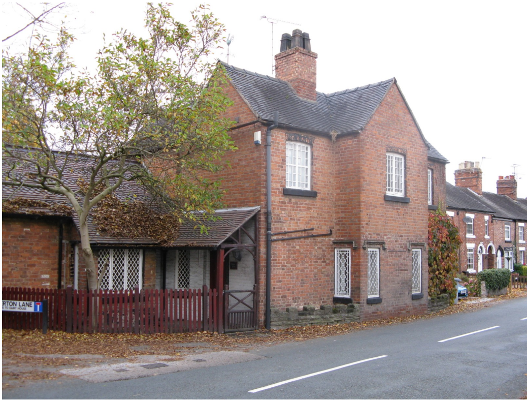
SJ 658 509. Audlem Road Tollhouse on A530. Whitchurch to Madeley Trust.
