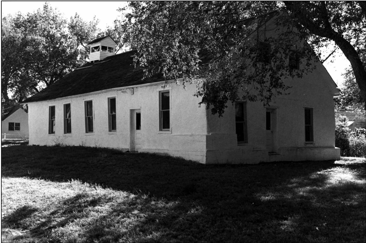
Photo 4 – north and east facades
