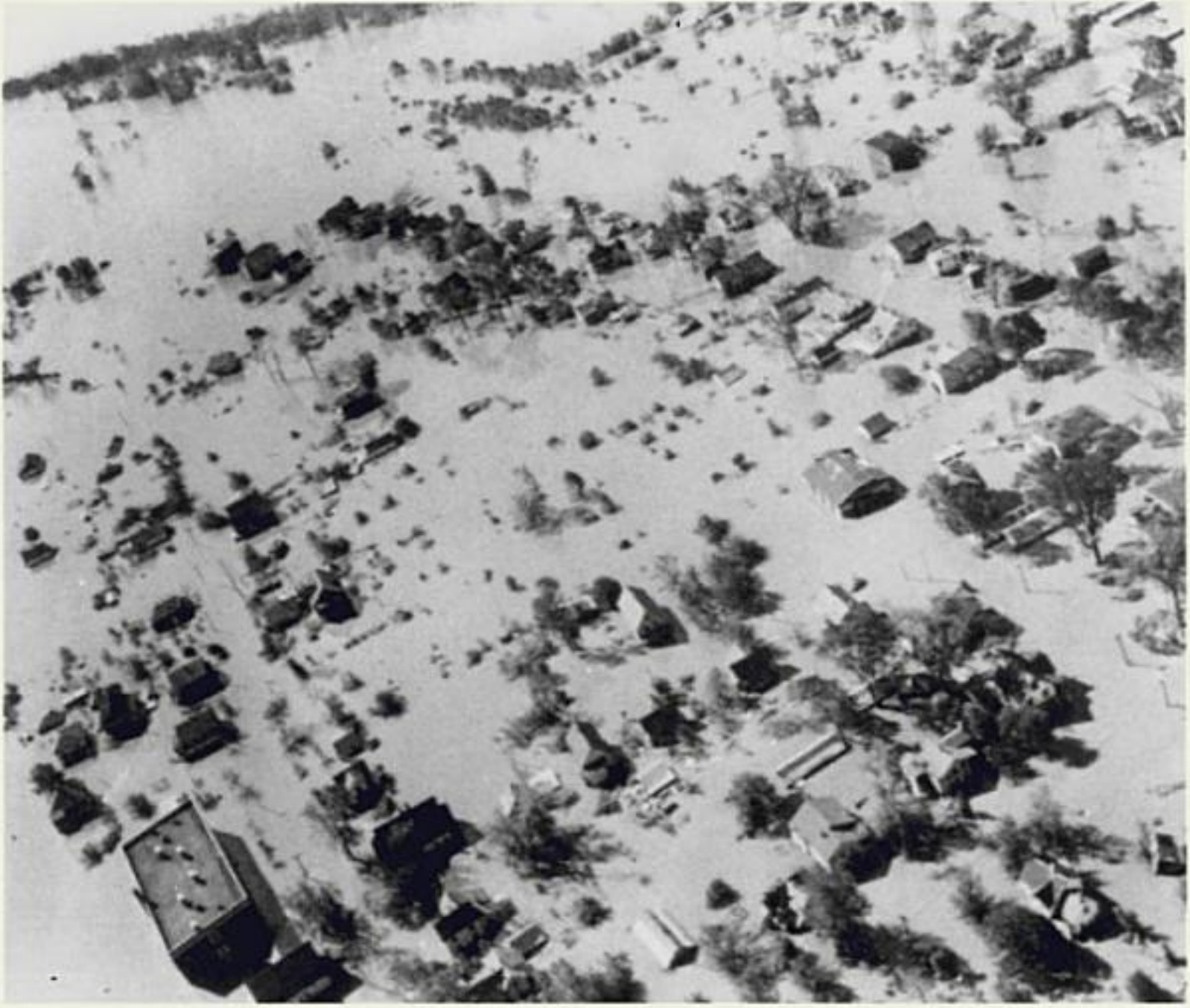
A flooded neighborhood in Hartford, Connecticut (courtesy of the Connecticut Historical Society)
