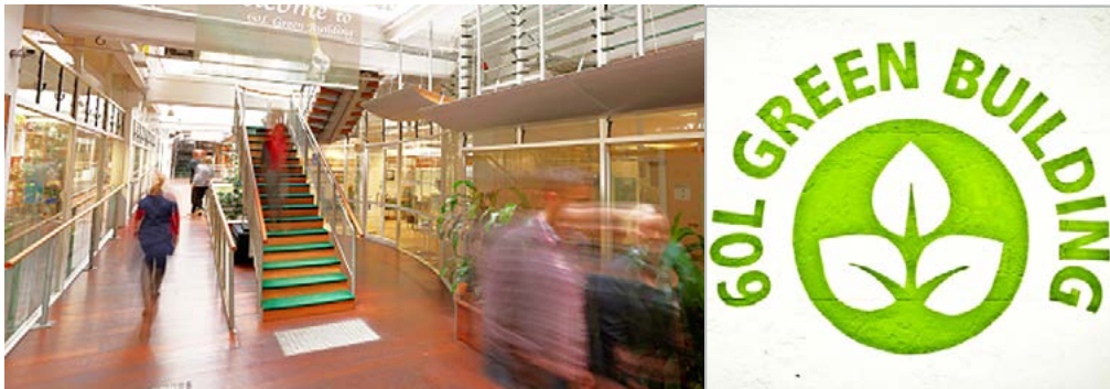
The 60L Green Building.
