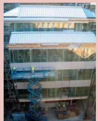
The North Courtyard building nears completion
