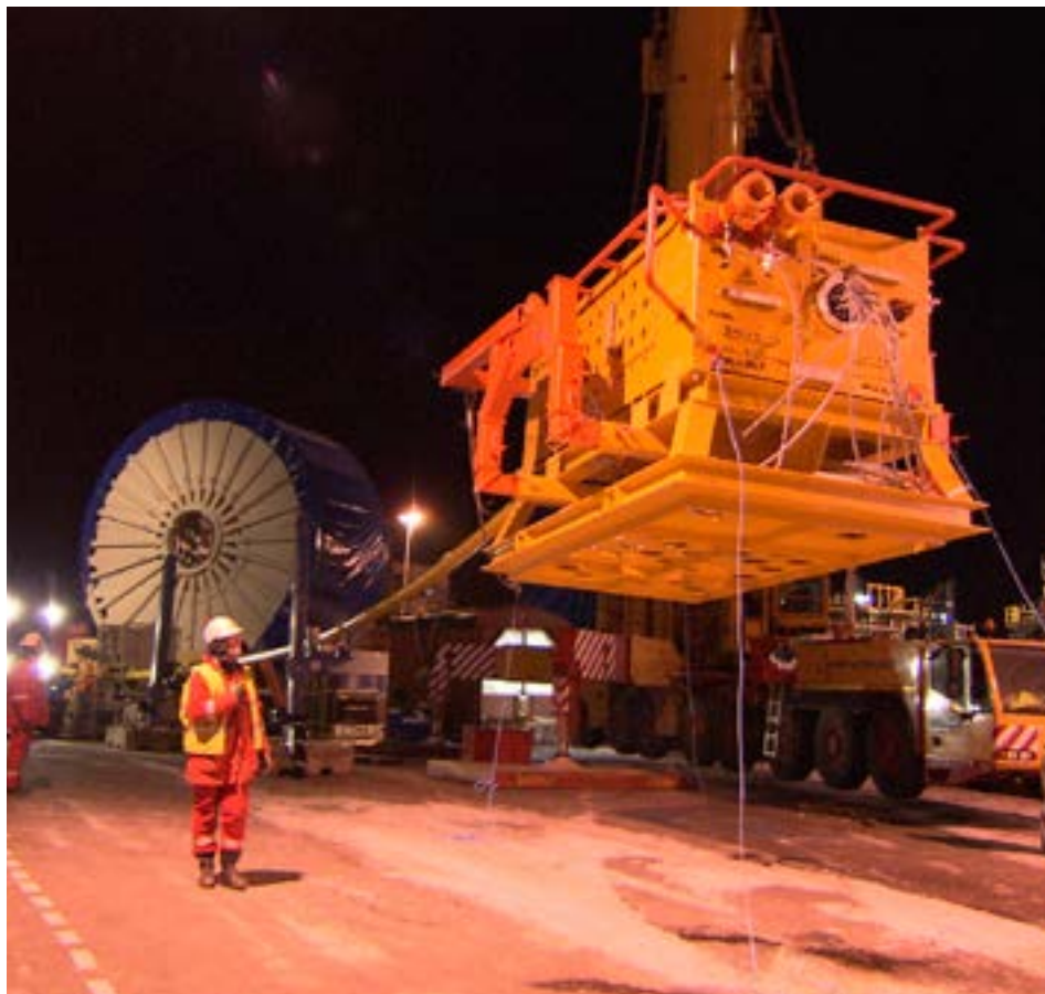
Subsea Distribution Units for the Jette field are loaded onto the Skandi Acergy in December 2012.
