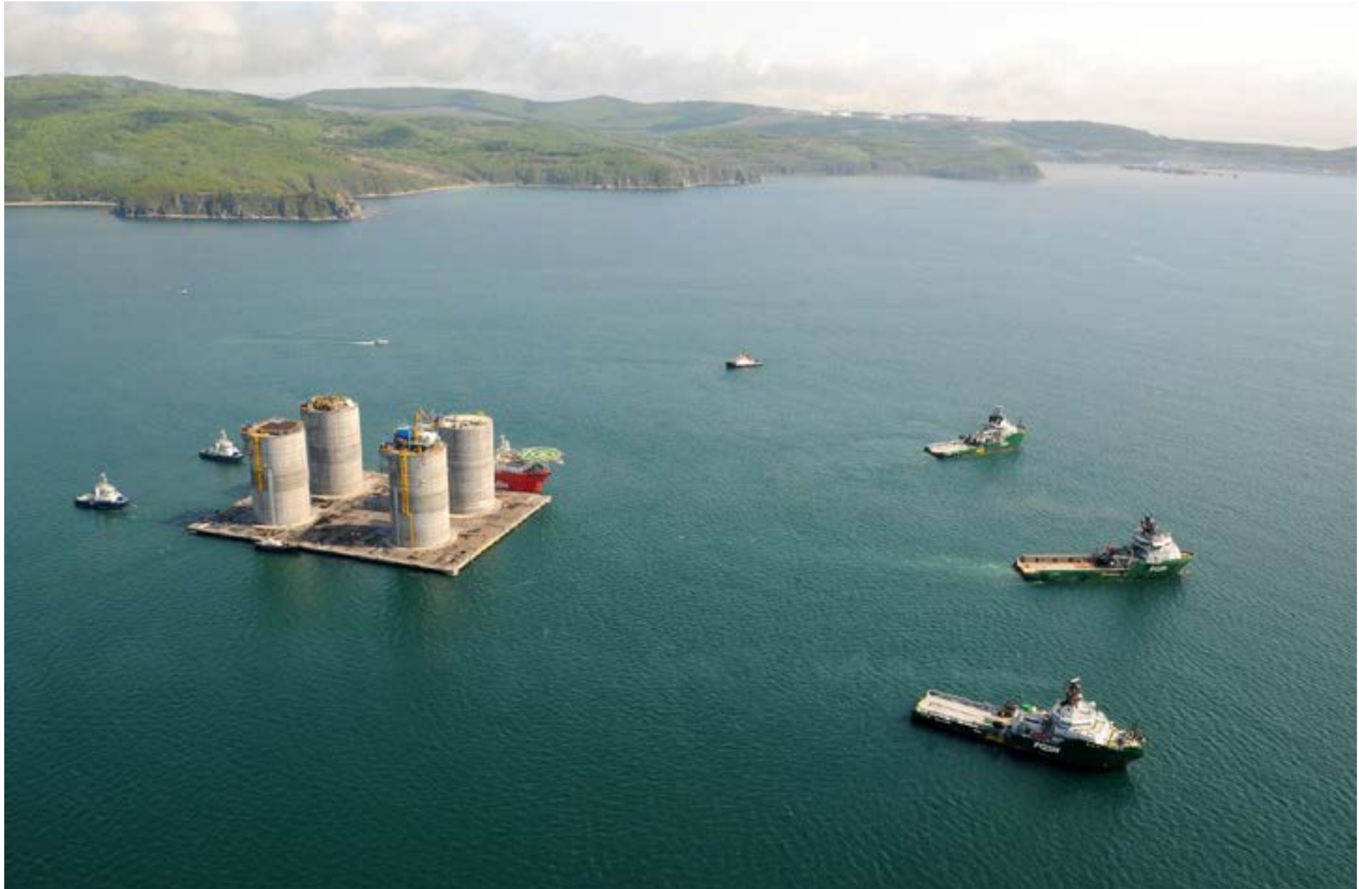
Kvaerner completes delivery: In 2012 the concrete substructure for Sakhalin I was towed and installed outside of the island carrying the same name.
