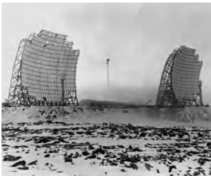
Figure 4-7 The 120 ft tropospheric scatter antennas at the Thule, Greenland, site. Snow coated the reflector screens during the winter.
