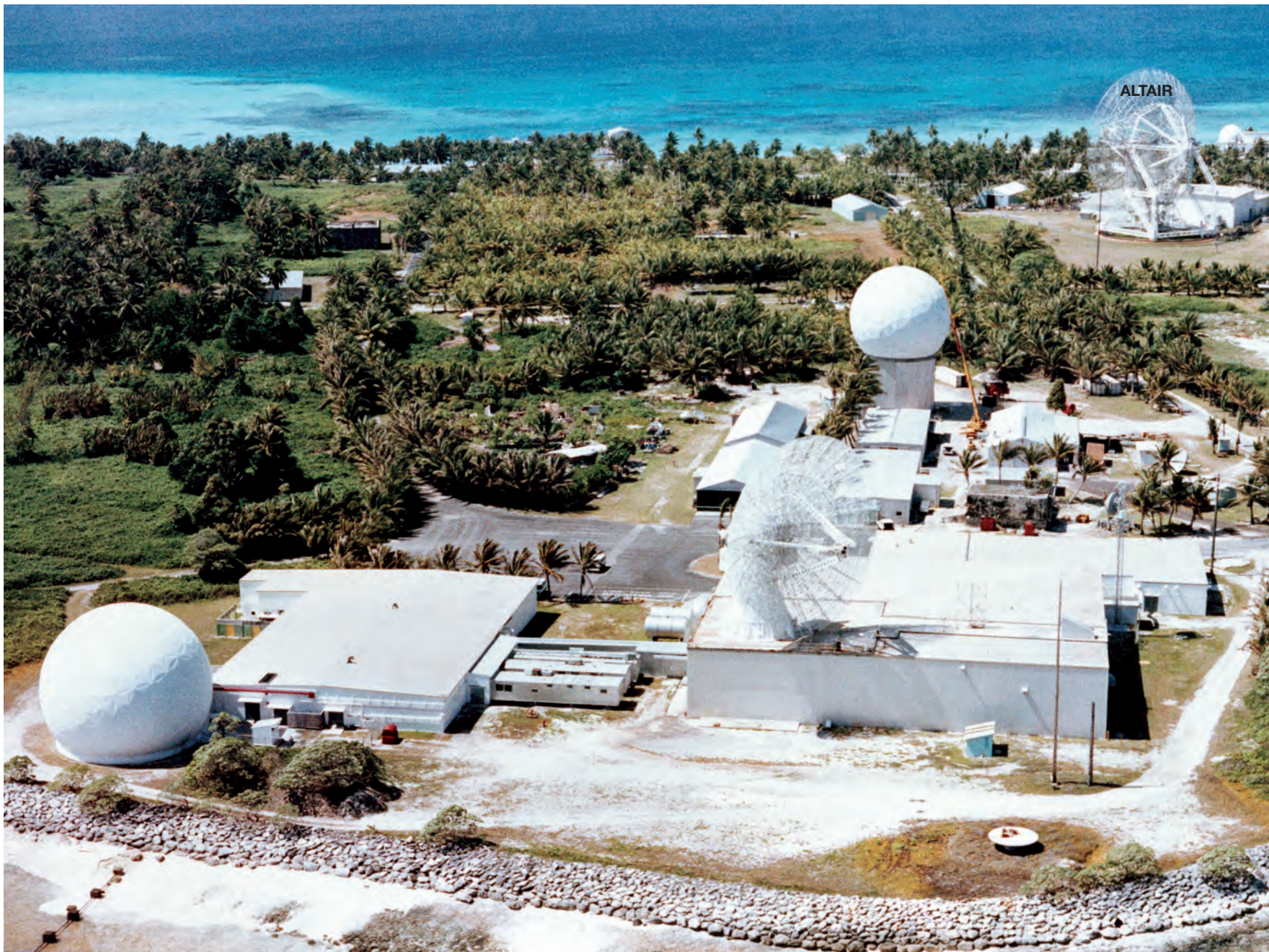
Figure 30-1 RTS instrumentation radars: ALCOR (front left), TRADEX (front right), MMW (center), and ALTAIR (back, near lagoon).
