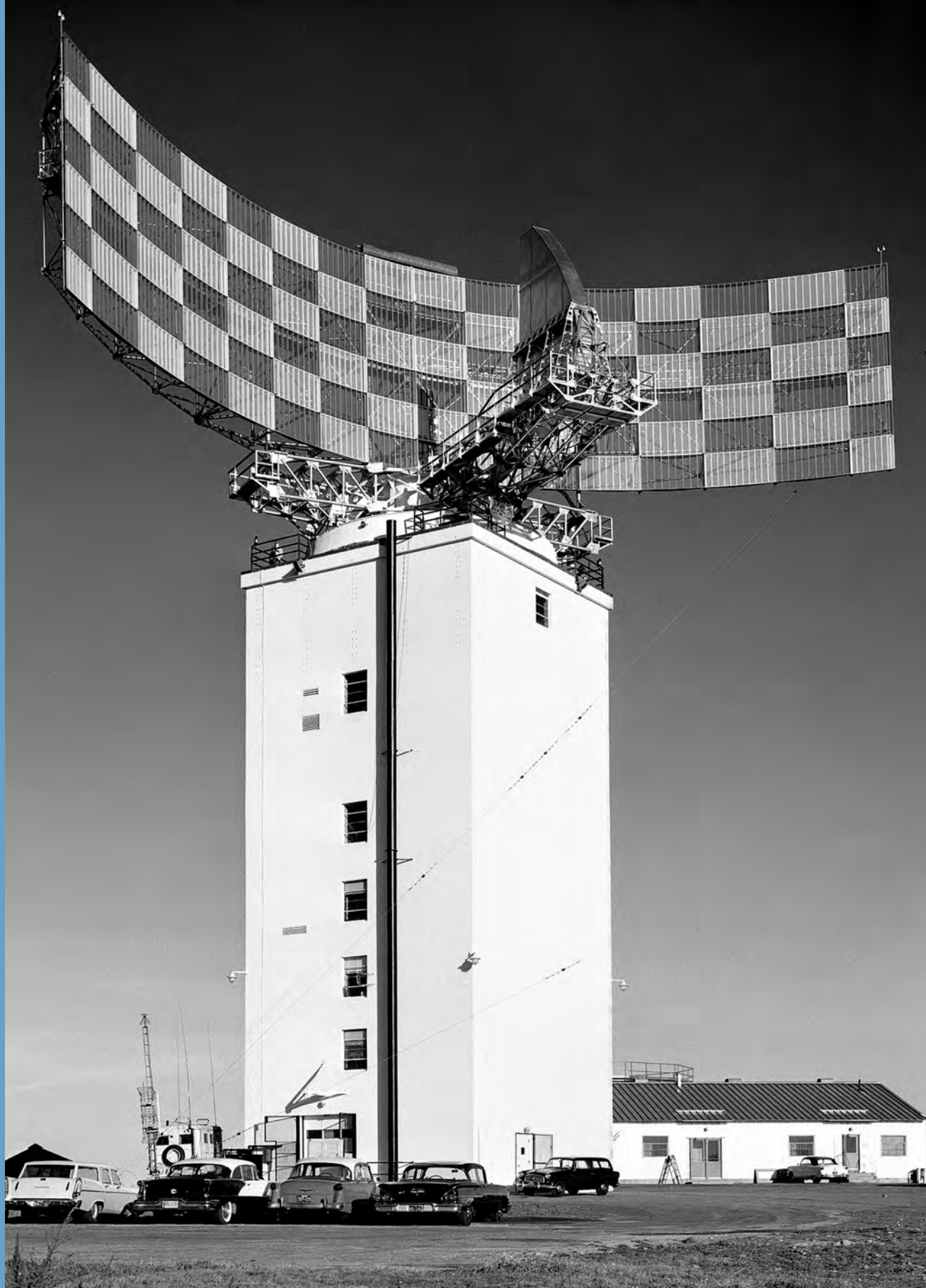
Figure 3-5 Boston Hill UHF GCI/CCM radar in North Andover, Massachusetts.
