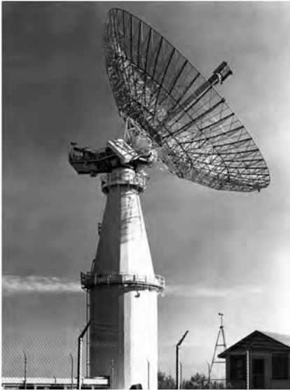
Figure 3-8 Antenna and supporting structure of the long-range UHF tracking radar on Millstone Hill in Westford, Massachusetts.
