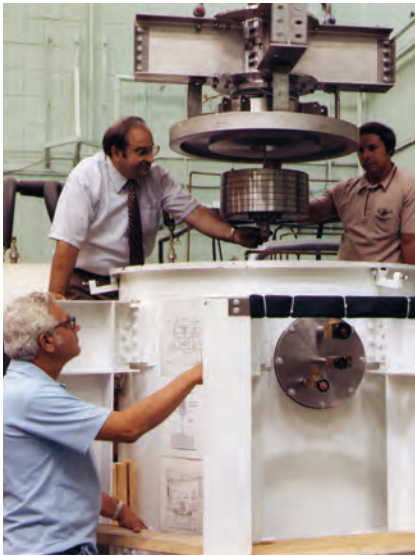
Figure 20-2 Charles Ciacera, Philip Jarvinen, and Frederick DiGregorio install a 1/10-scale flywheel system to evaluate the feasibility of a kinetic-energy storage proposal.
