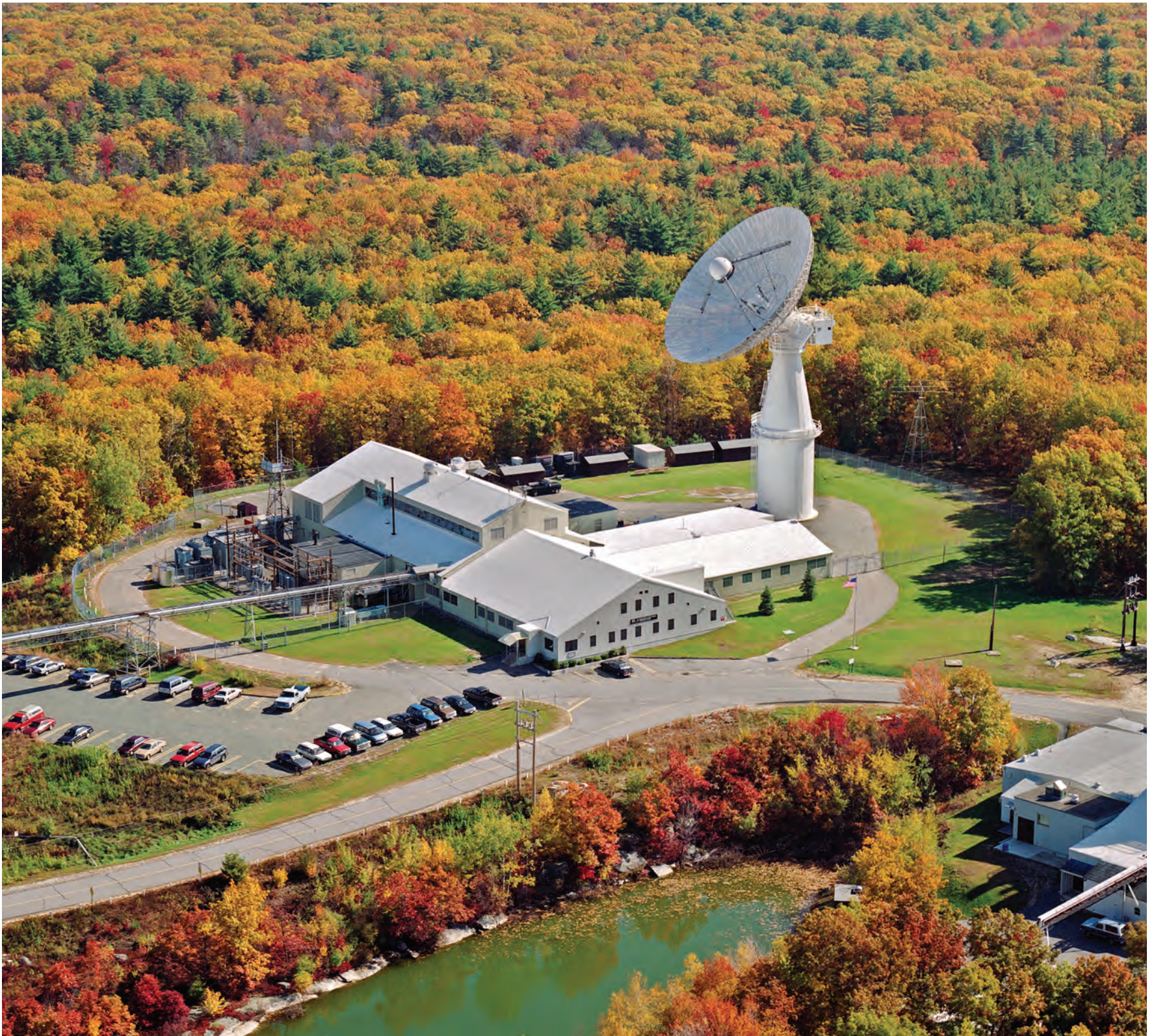
Figure 10-2 Millstone radar with 84 ft antenna.
