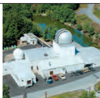
Firepond Laser Radar Facility, Westford, Mass.
