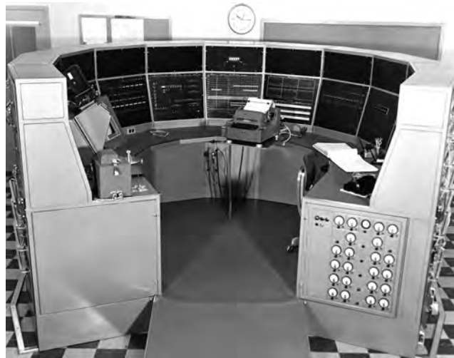
Figure 28-4 CG-24, the first all-transistor computer.
