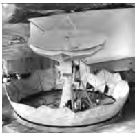
Construction of ALCOR, Roi-Namur
