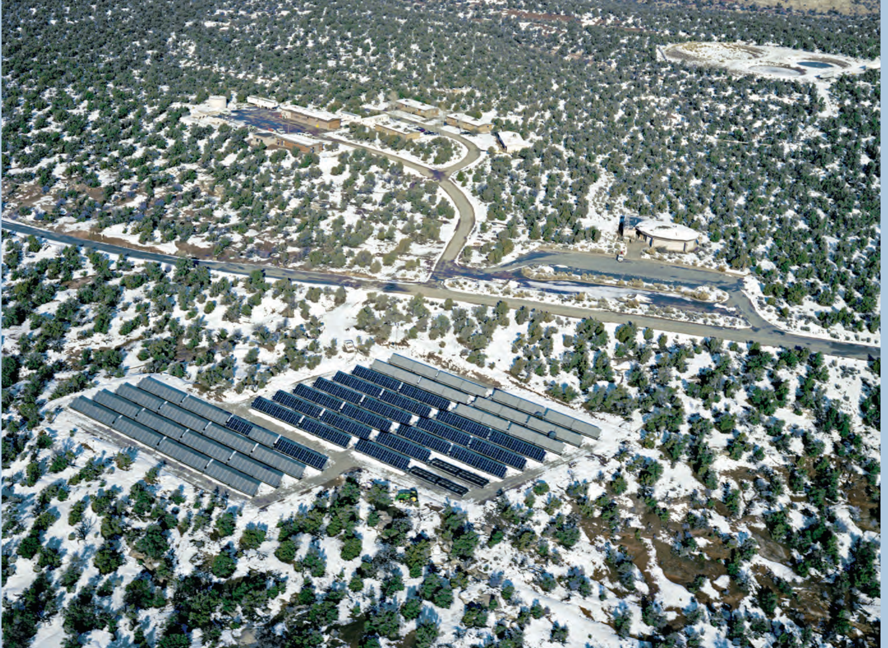
Figure 20-1 Solar-photovoltaic power station at Natural Bridges National Monument, Utah.
