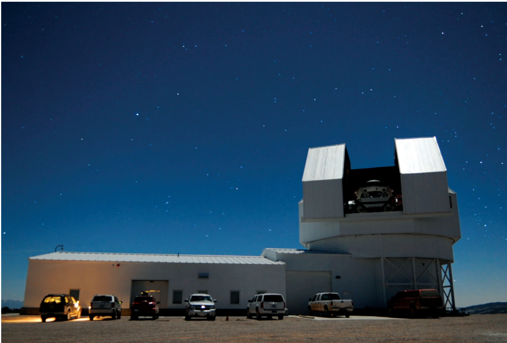
Figure 10-15 The enclosure for the SST under construction near North Oscura Peak on the White Sands Missile Range. The enclosure incorporates state-of-the-art techniques and cooling to preserve the pristine observing conditions found at the site and to allow SST to achieve its full potential.
