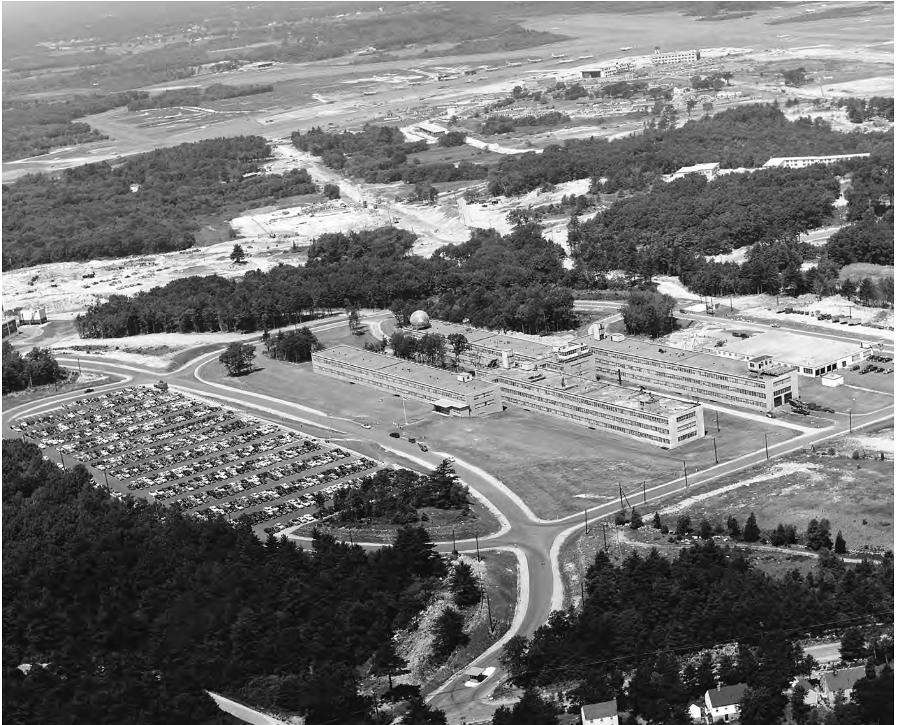
Figure 1-8 Original Lincoln Laboratory building complex in Lexington.
