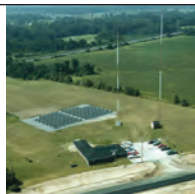
Radio station WBNO photovoltaic-powered transmitter site, Bryan, Ohio
