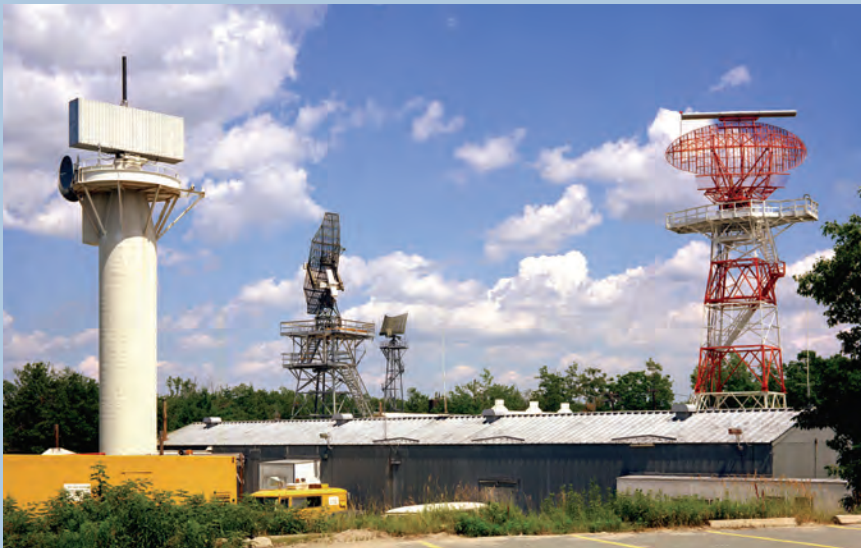
Figure 12-1 DABS/Mode S experimental facility with two experimental radars in the background.
