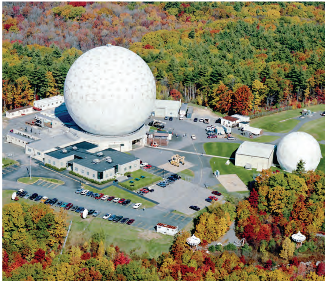
Figure 10-6 Haystack radar site. The LRIR Haystack antenna is in the large radome on the left; the HAX radome and equipment building are on the right. HAX was completed in 1993 to collect satellite-imaging and space-debris data.
