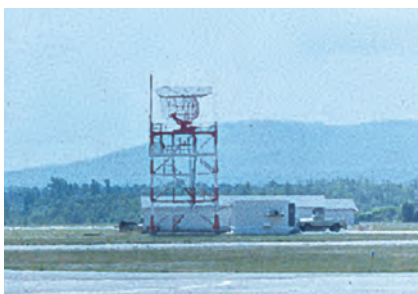
Figure 12-4 Airport surveillance radar with Lincoln Laboratory-developed MTD processor in Burlington, Vermont. The surrounding hills provided a high-clutter environment to test and demonstrate the clutter-reduction capability of the radar.
