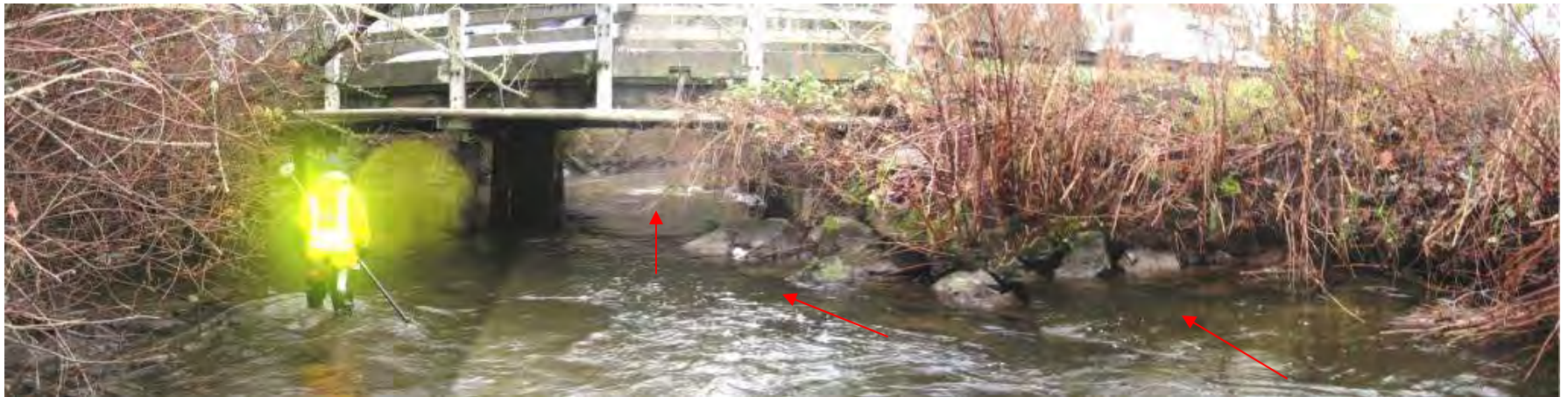
Figure 4. View looking downstream toward Union River bridge.
