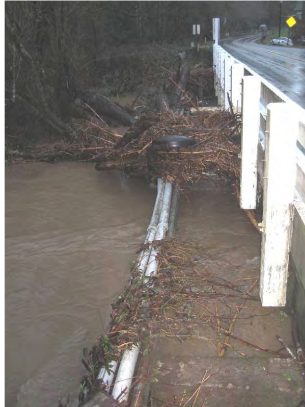
Figure 5. Wood debris on upstream side of Union River Bridge. Note utility conduit paralleling the bridge.
