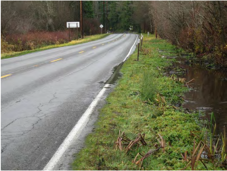
Figure 10. Ditch along north side of SR 300 in the wetland section.
