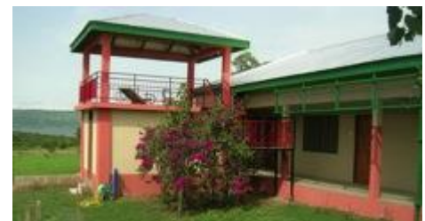
View of part of the rectory at Ekye
