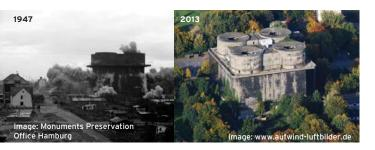
In 1947 the building's interior was blown up by the British army. Six of the building's eight storeys collapsed and the remaining structure became too unsafe for people to enter. The outer shell with up to three metres thick walls and up to four metres thick floors was all that remained relatively undamaged. For over 60 years it was inconceivable that a new use would be found for the whole building, except for some ancillary uses in parts of it.
