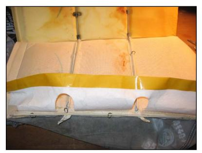
Take off the adhesive-covering strips at the ends of the element inside the sleeves and attach to the fleece.
