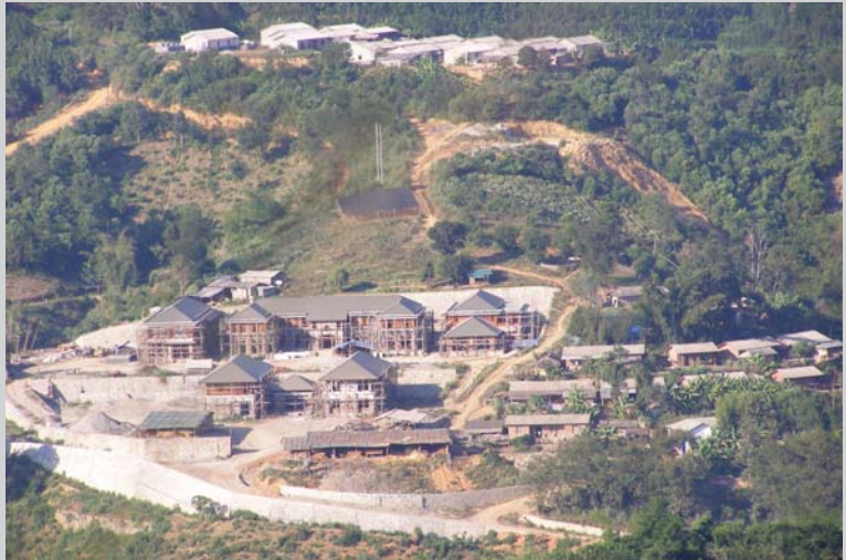
Wei's new mansion and Hong Pang offices at Wan Korng, 3-4 kms west of Panghsang, under construction since 2005 at a cost of 200 million yuan (nearly 1 billion baht)
