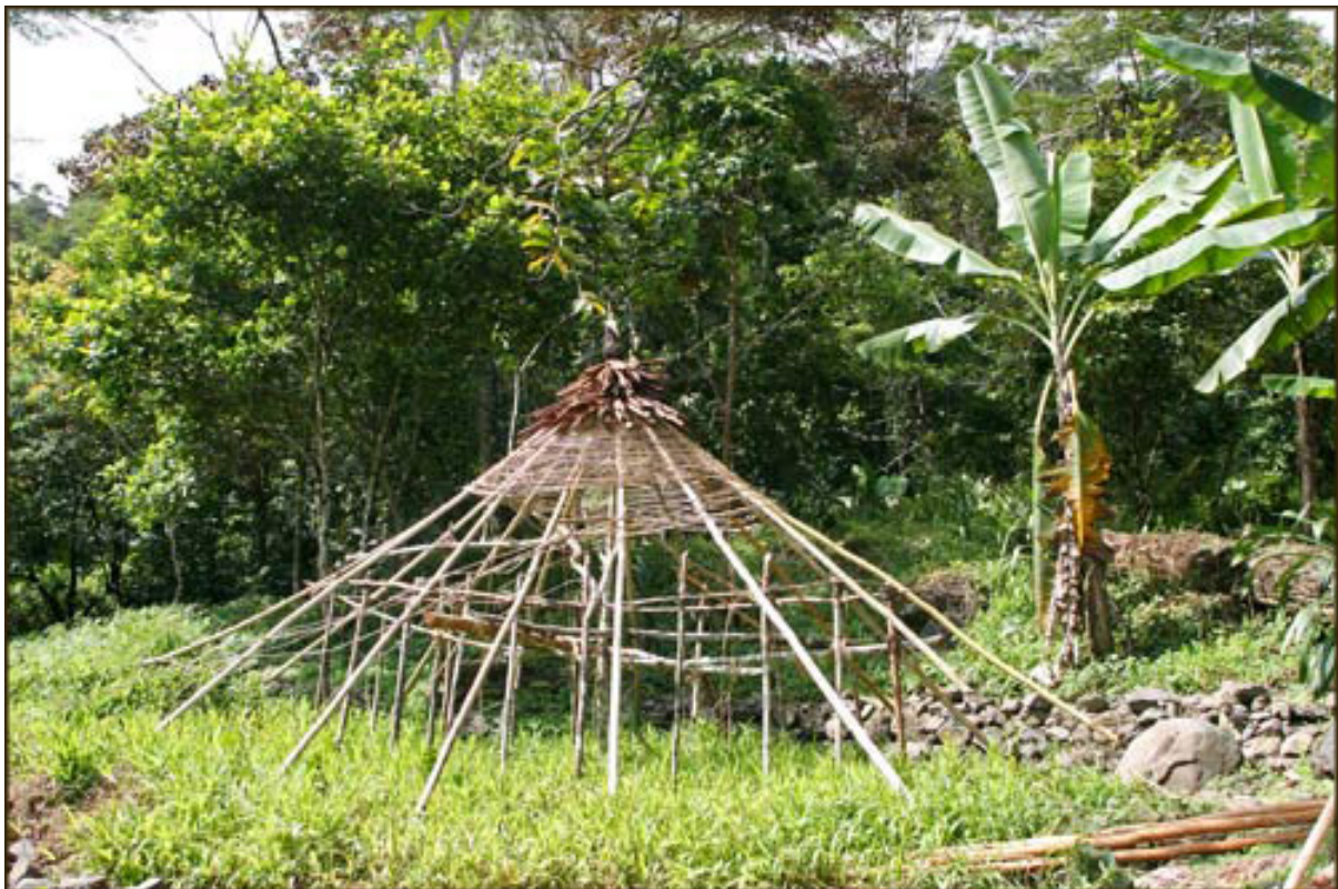
New hut in process of being built
