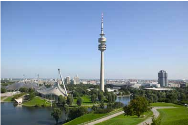
Communication tower in city
