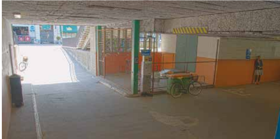
Figure 11: Parking garage, indoor. The image is taken from an Axis camera that incorporates the WDR-dynamic capture technology.
