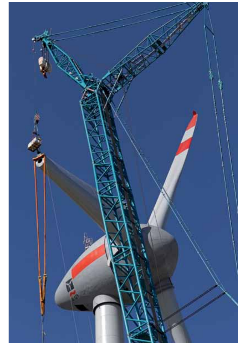
Rotor blade assembly on ENERCON E-126 turbine at WKA Project.
