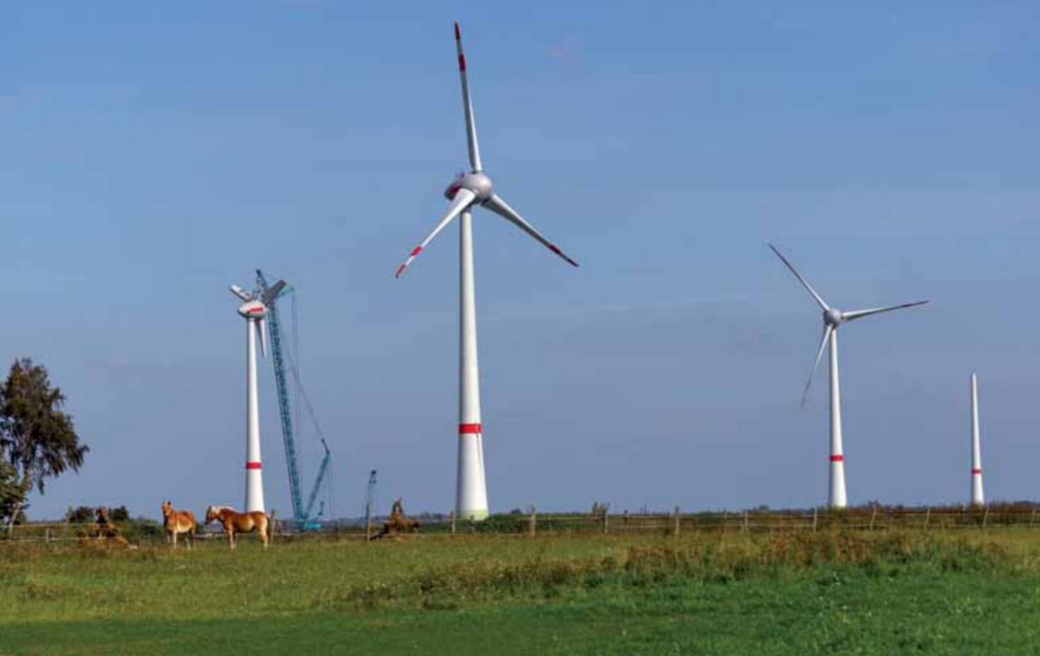
Multi-megawatt turbines under construction: ENERCON E-126/7.5 MW at WKA Project.
