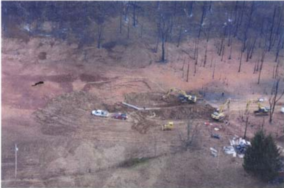
Figure 2. Aerial Photograph of Failure Site
