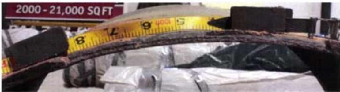
Figure 4. Photograph of the fracture surface from Failed Girth Weld Section (U/S) from approximately 0 to 1 foot clockwise (looking D/S) of TDC.
