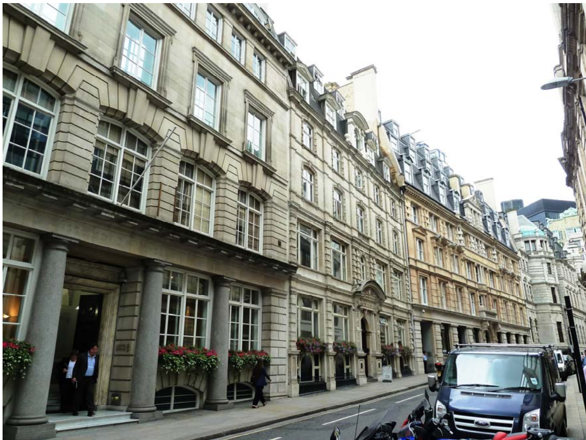
Lloyd's Avenue, west side
