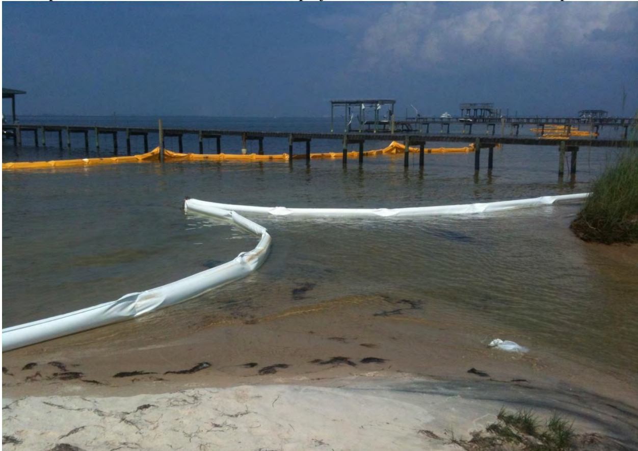
Figure 4. The City of Gulf Breeze West Side Protection Project and the three tier protection boom of Zamara Canal. Both protection strategies impede potential wetland breaching of oil.
