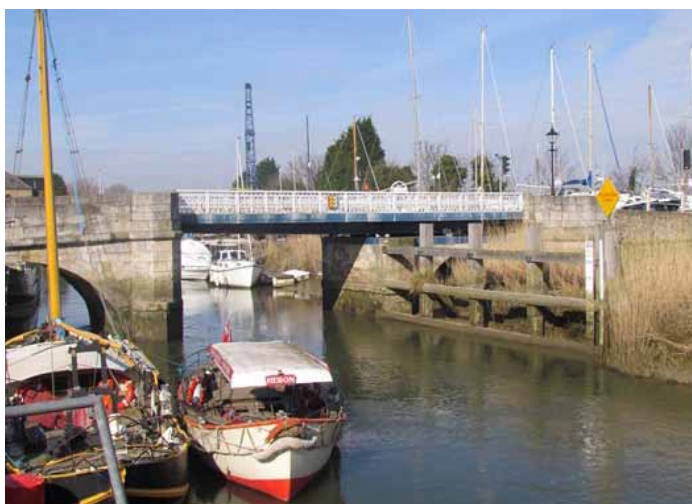
The town bridge was rebuilt using funds raised by the tolls Rory Walsh © RGS-IBG Discovering Britain
