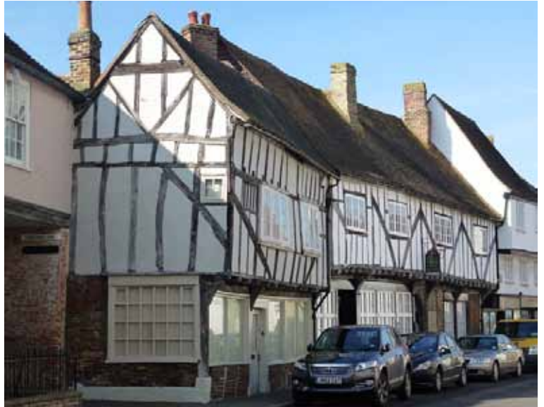
Timber frame buildings in Strand Street Rory Walsh © RGS-IBG Discovering Britain
