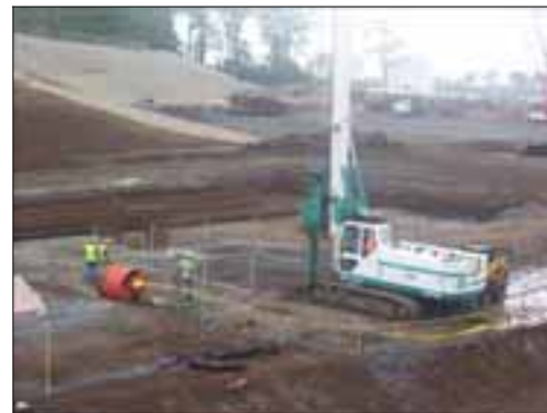
Drilled Shaft Drilling Machine
