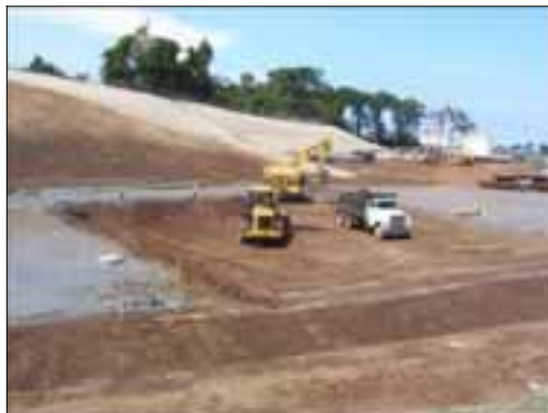
Preparing Land Tower Foundation Site
