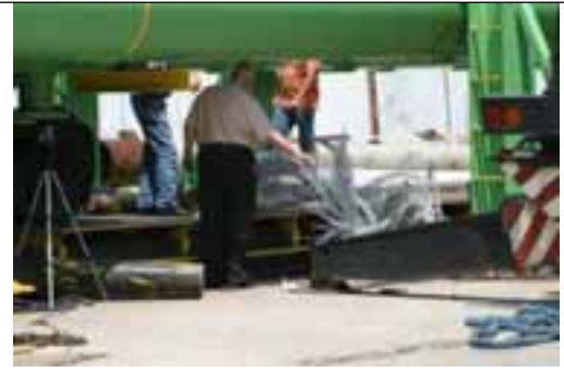
Main Strand After Load To Fail Test
