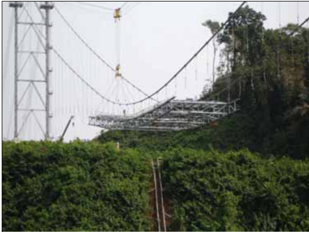
First Six Deck Modules Installed
