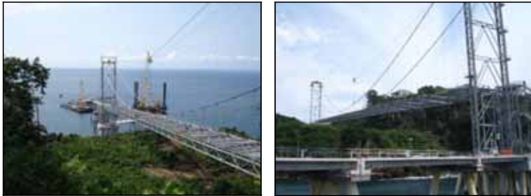
All Deck Modules Installed
