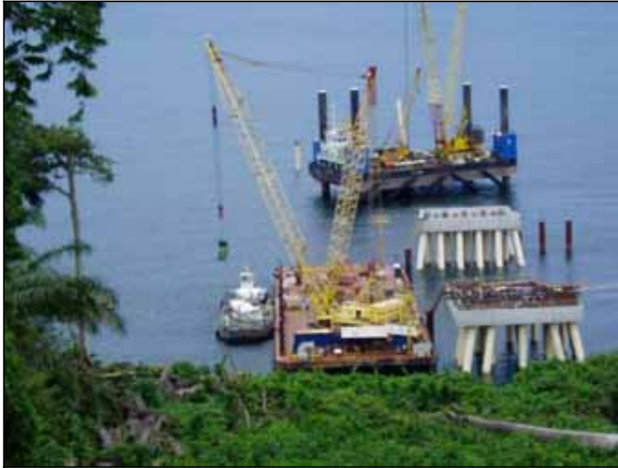
Placing Concrete For Marine Tower Pile Cap
