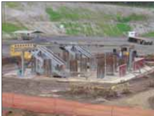
Land Anchor Embedments Placed
