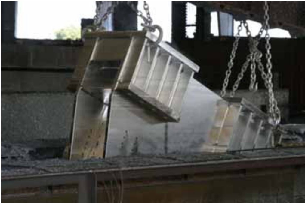
Freshly Galvanized Tower Base Section Lifted From Molten Zinc Bath
