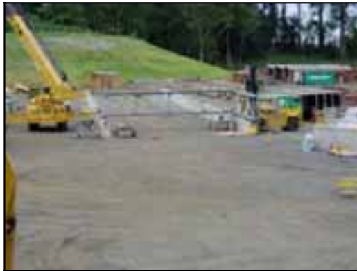
Deck Module Assemble Begins
