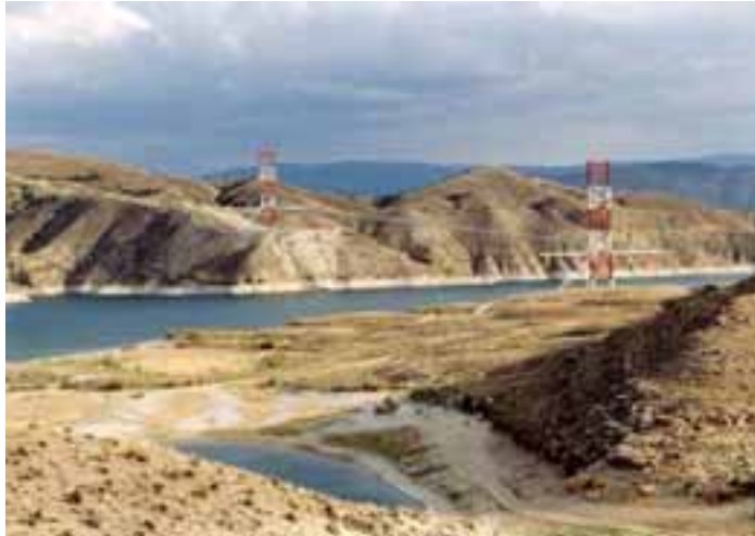
Cable Pipeline Bridge – Flaming River, Wyoming, USA
