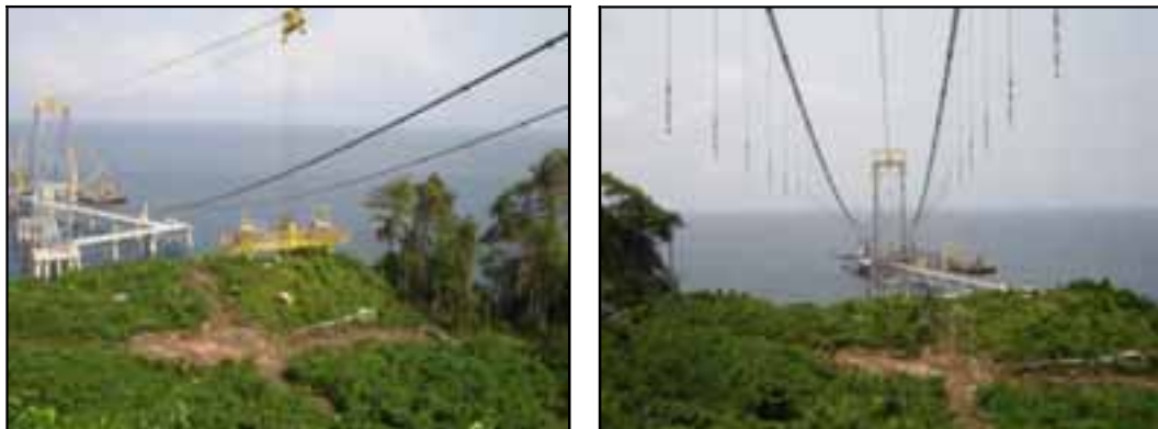
Hanging Suspender Wires
