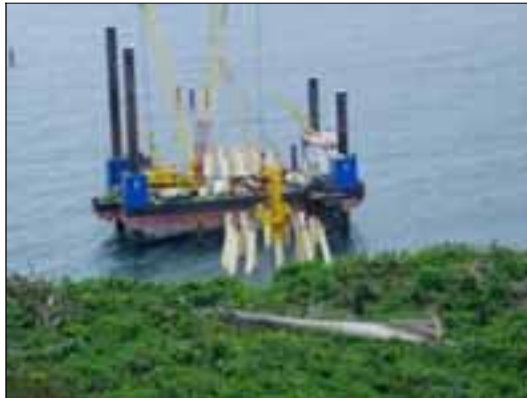
Drilling Pile for Marine Tower Foundation
