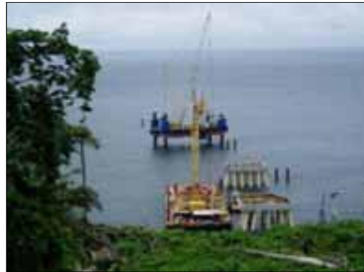
Placing Reinforcing Steel For Marine Tower Pile Cap
