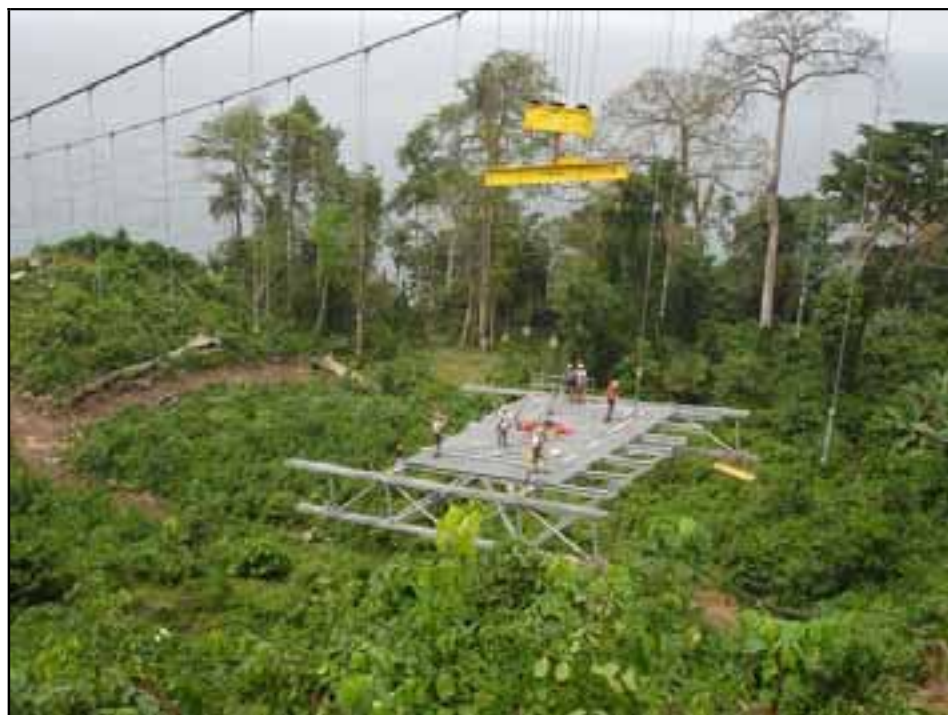
First Deck Module Transported by Highline
