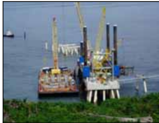
First Section of Marine Tower Erected
