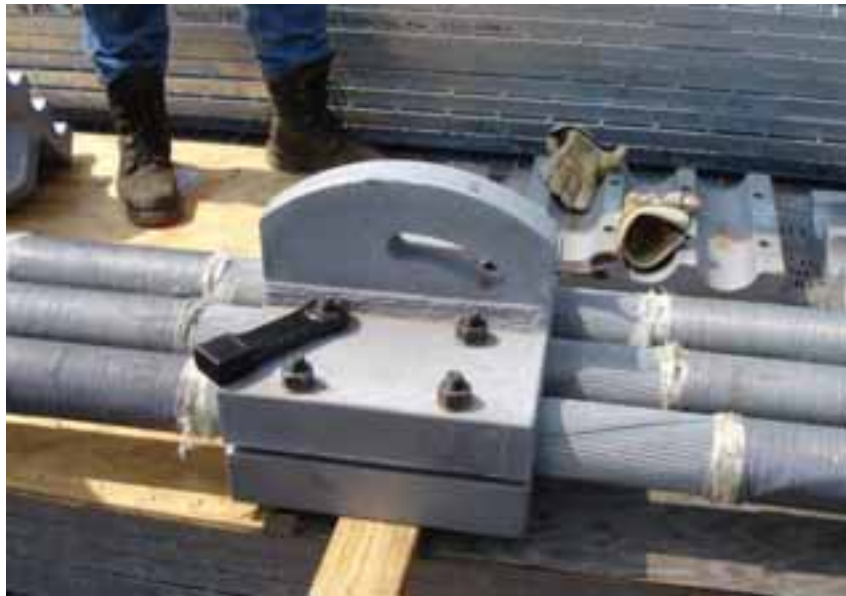
Cable Clamp Trial Fit
