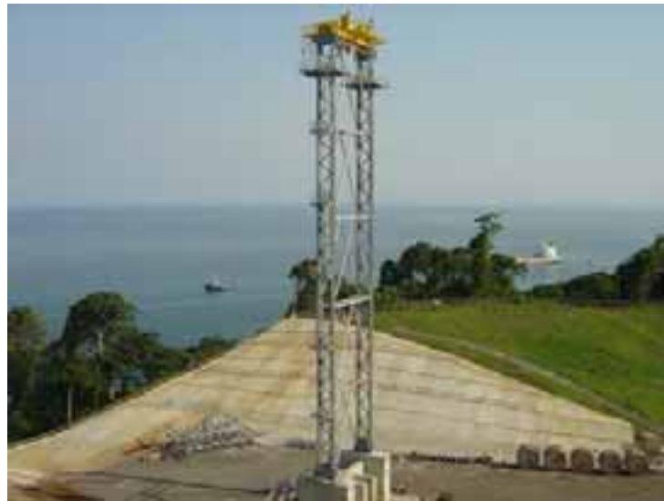
Land Tower Erection Complete with Temporary Equipment Deck
