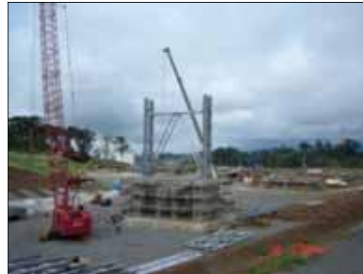
First Bent of Land Tower Erected
