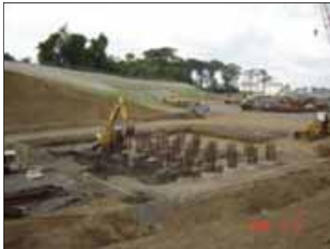
Land Tower Drill Shafts Complete
