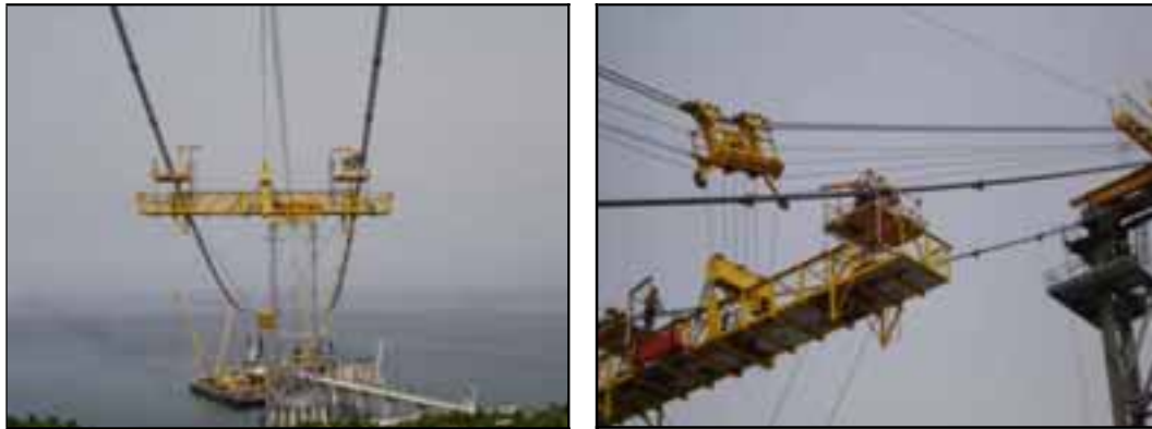
Installing Cable Clamps on Main Strand
