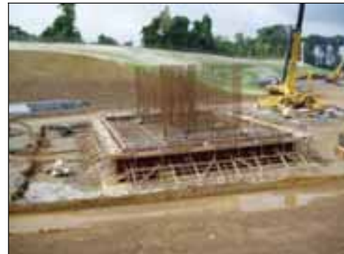
Land Tower Pile Cap and Pedestal Steel
