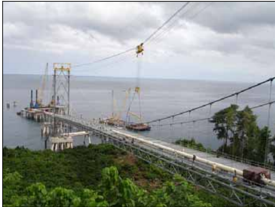
Pipe Installation with Highline
