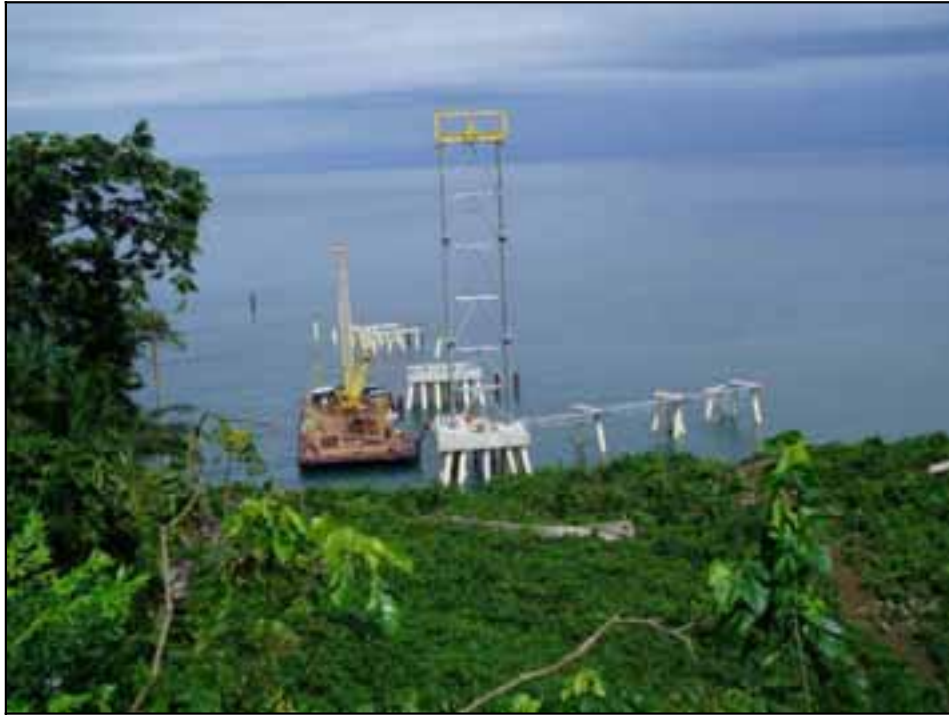
Marine Tower Completely Erected
