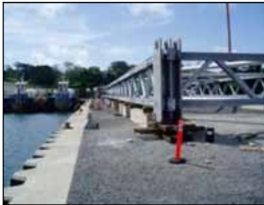
Marine Tower Test Assembly at Construction Jetty
