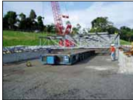
Completed Deck Module
