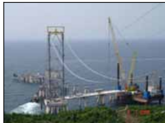
Main Cables Installed
