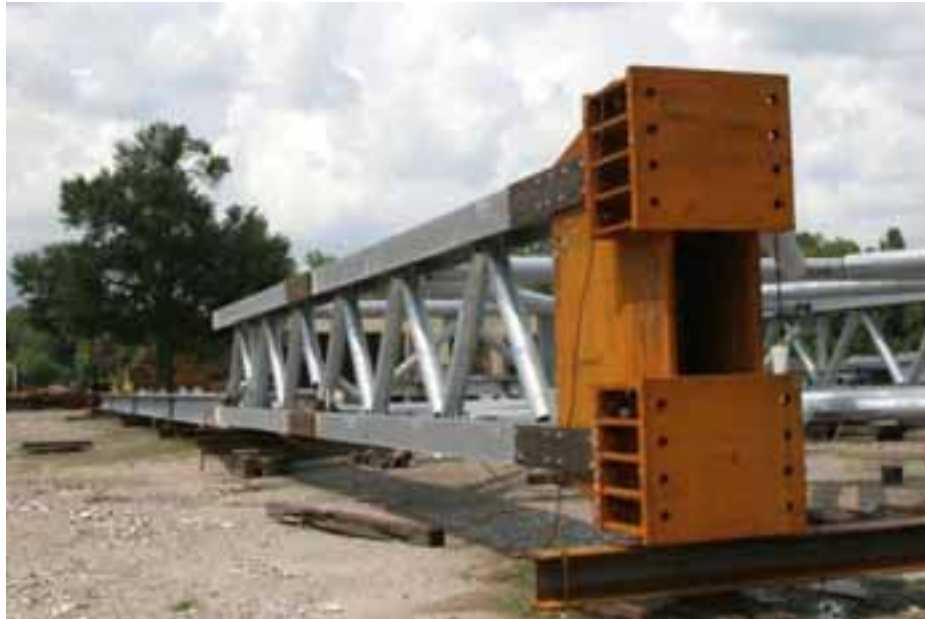
Trial Assembly of Marine Tower
