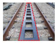
In addition to the earthquake resistance reinforcement of bridge piers and stations, we are moving forward with the installation of derailment prevention quards for Shinkansen.
