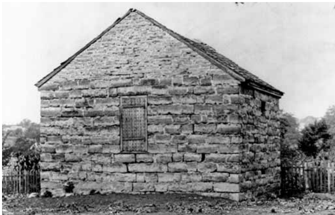
Liberty Jail. The Prophet Joseph and several other Church leaders were confined in a cold, dark, dirty, fourteen-foot-square cellar room of the jail called the “dungeon.” The outer walls of the jail were gray limestone rock and two feet thick, with a sturdy inner wall of hewn oak timbers. The jail was constructed in 1833 and was used for twenty-three years.
