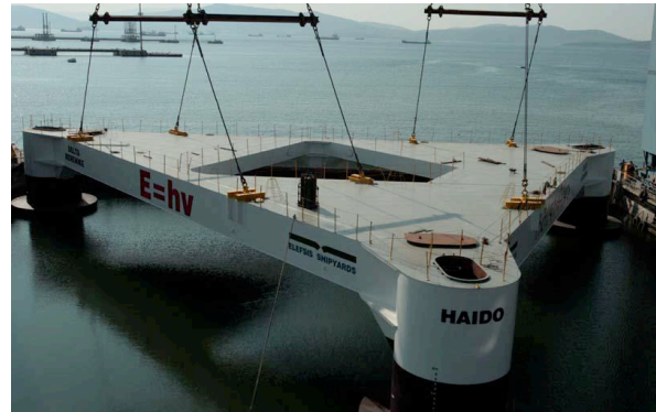
Figure 3-48: Surface platform “Delta Vereniki” Left: Mechanical drawing of girder structure; Right: Photo during launch.
