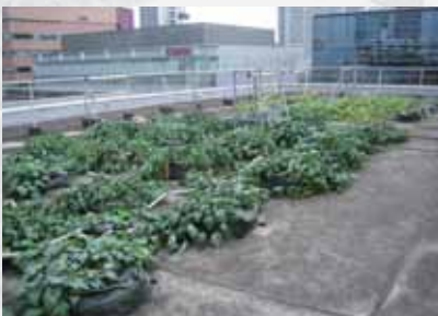
Rooftop greening to increase urban green space (growing sweet potatoes) (NTT URBAN DEVELOPMENT and NTT FACILITIES)
