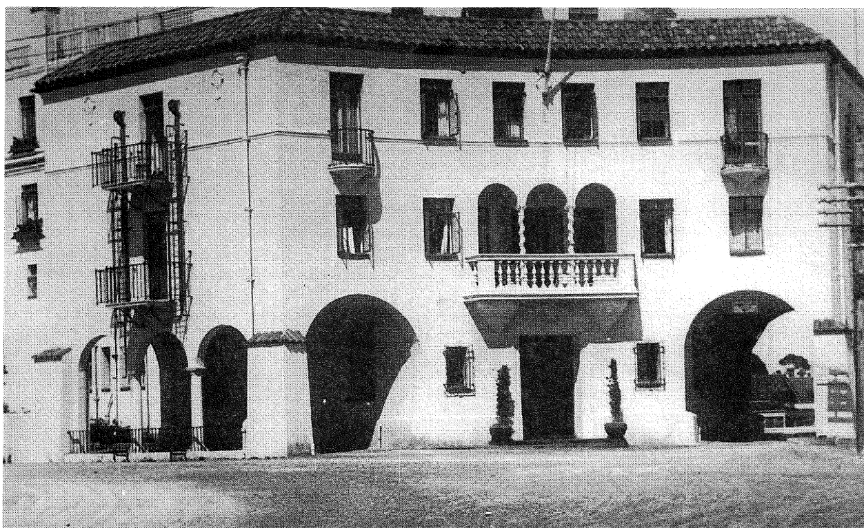
Figure 11: (b) A poor reinforced concrete building. The Nurses' Home at Napier Hospital before the earthquake, the only r.c. building to collapse completely, due to a bottom storey weakened by large openings and little reinforcement (Courtesy of the Alexander Turnbull Library, Wellington).
