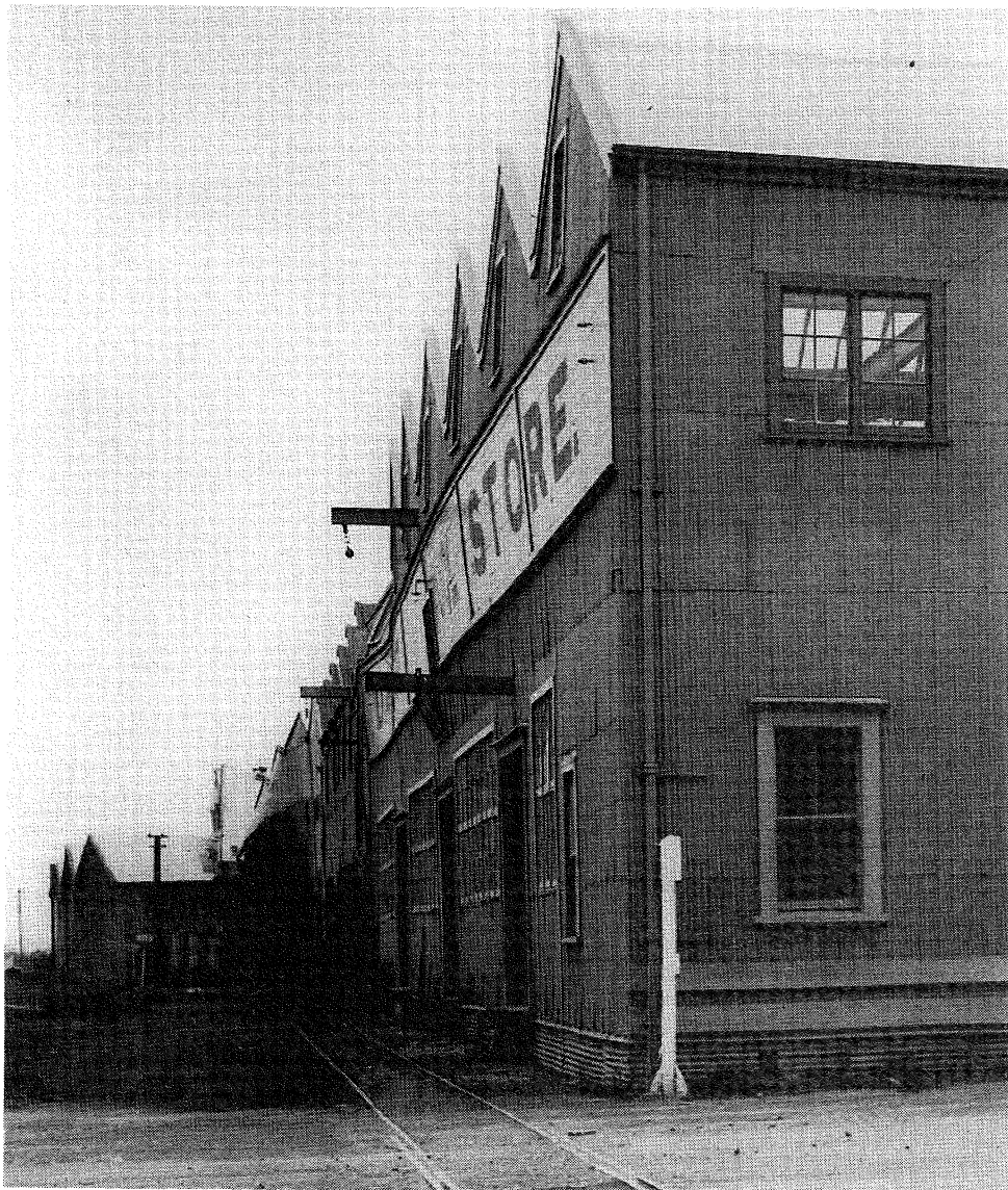
Figure 10: Dalgety's No. 2 Store, Port Ahuriri, Napier one of the few steel-framed buildings in the region, was inadequately braced. (Courtesy of the Alexander Turnbull Library, Insurance Council of NZ Collection, Wellington).
