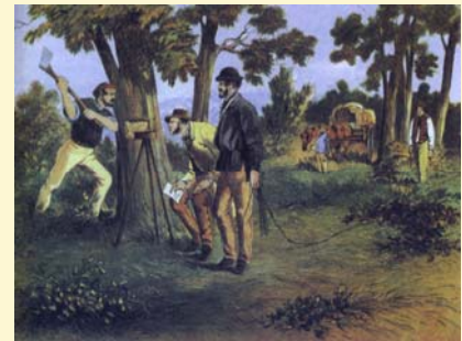
Surveyors by S.T. Gill (State Library of Victoria). A survey party at work using a circumferenter and chain and blazing a tree to mark a line. This was the method used by MacCabe on the river surveys.
