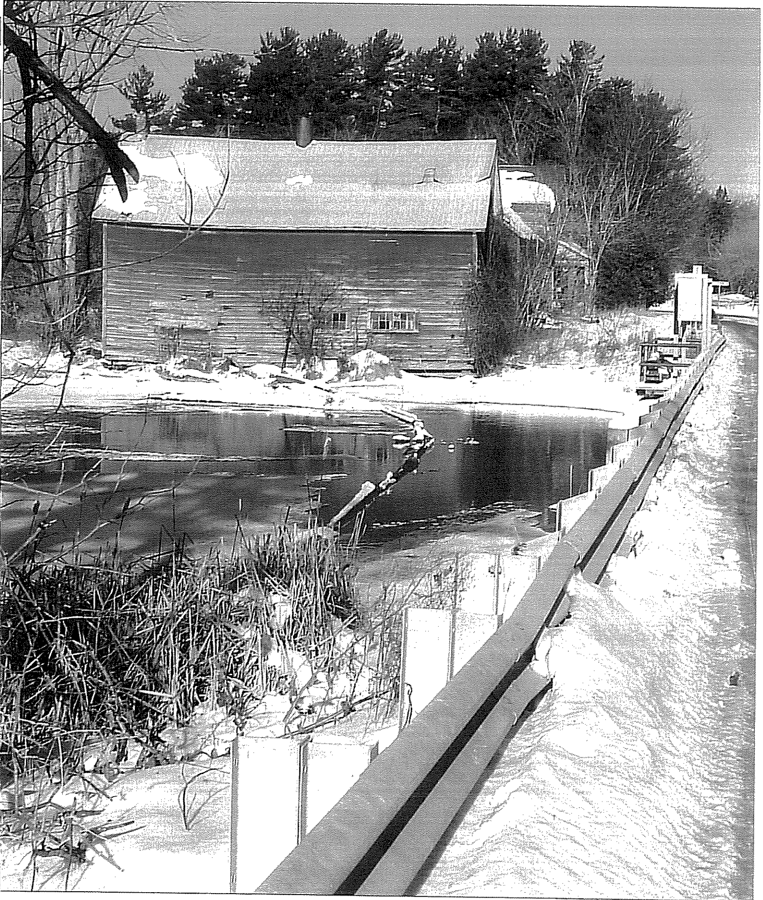
Figure 10: Photograph of the upstream construction area
