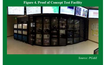
Ancillary equipment is the hardware required to support PMU operation, apart from the PMU itself. Such equipment includes GPS clocks, PDCs, network switches and routers, cabinets and computers. The cost of this equipment is generally low relative to the installed cost.
