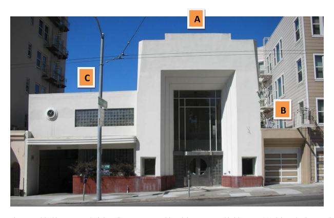
The original building consisted of the tall center structural bay (A), a garage added later in 1932 (B), and a horizontal addition in 1940 (C).
