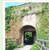
When the B&ER was being built in the early 1840s the meander at Bathpool was bypassed by diverting the Tone into a new channel (the "New Cut") alongside the railway line, thus eliminating the need for two railway bridges over the river. Brunel's assistant, William Gravatt, designed three arches to carry the Bridgwater road on a skew angle over the river, the towpath and the railway. Over the New Cut
