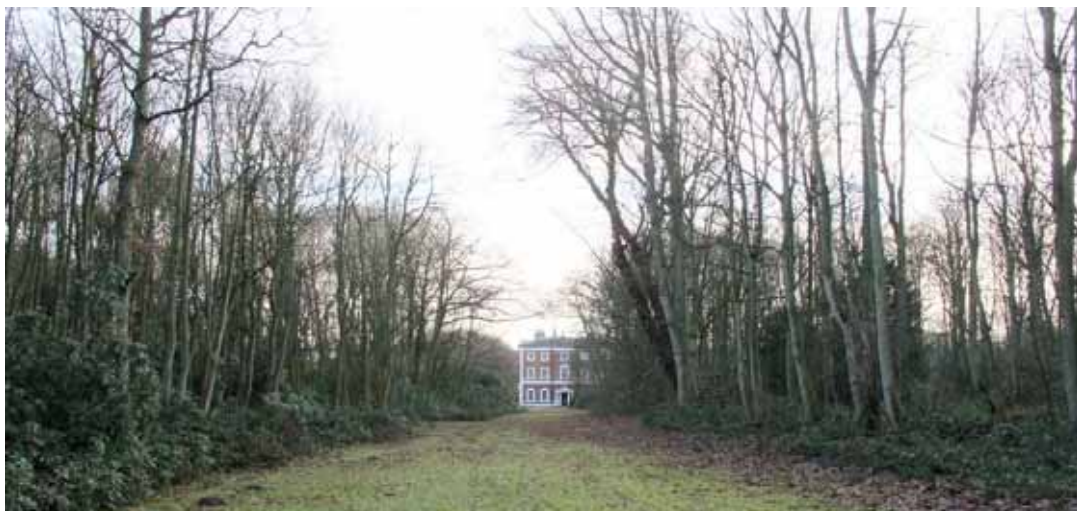
Figure 7: The North Prospect: encroaching sycamore and Rhododendron to be removed
