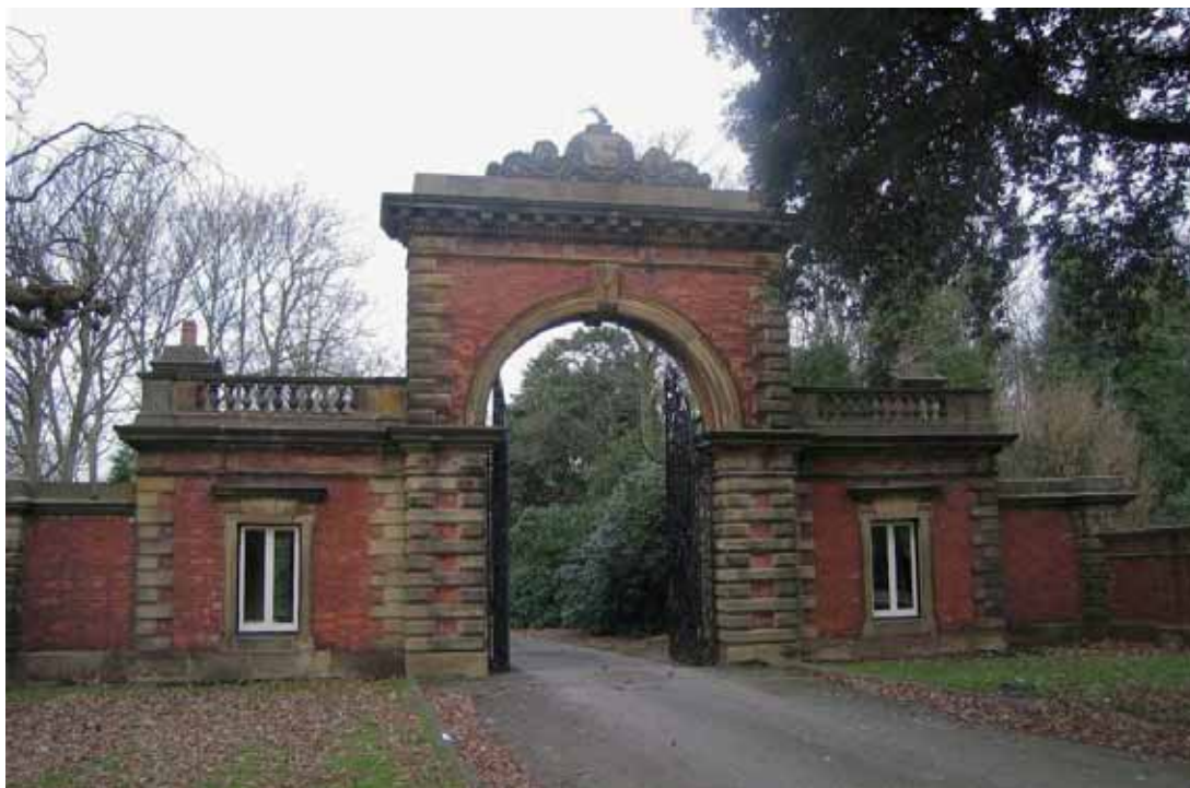
Figure 39: A new path from the Main Lodge to the Inner Gate is proposed, to separate pedestrian and vehicular traffic
