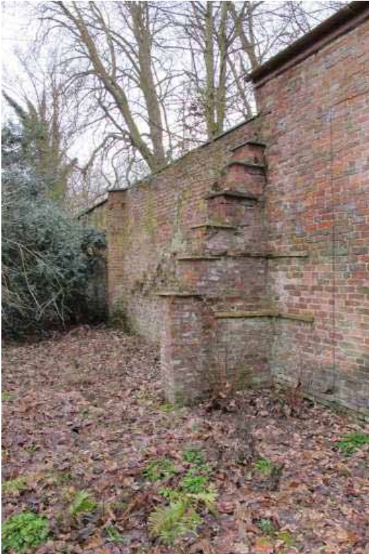
Figures 59 to 63: The historic garden wall (above and below) will be repointed. Small areas of modern brick will be replaced, and modern coping will be replaced with brick coping to match the surviving length of the original detail.
