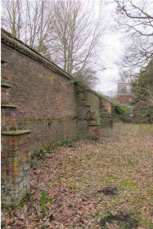
Figures 59 to 63: The historic garden wall (above and below) will be repointed. Small areas of modern brick will be replaced, and modern coping will be replaced with brick coping to match the surviving length of the original detail.
