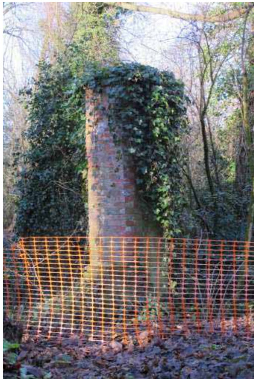
Figures 59 to 63: The historic garden wall (above and below) will be repointed. Small areas of modern brick will be replaced, and modern coping will be replaced with brick coping to match the surviving length of the original detail.
