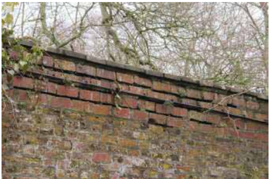
Figures 59 to 63: The historic garden wall (above and below) will be repointed. Small areas of modern brick will be replaced, and modern coping will be replaced with brick coping to match the surviving length of the original detail.
