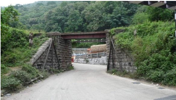
Railway Line , bridges and road
