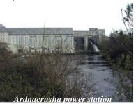
400m<sup>3</sup>sec<sup>-1</sup> water supply needed for maximum generation levels. A 2.4 km long tailrace canal returns the station discharge back to the River Shannon. The Parteen regulating weir, located
