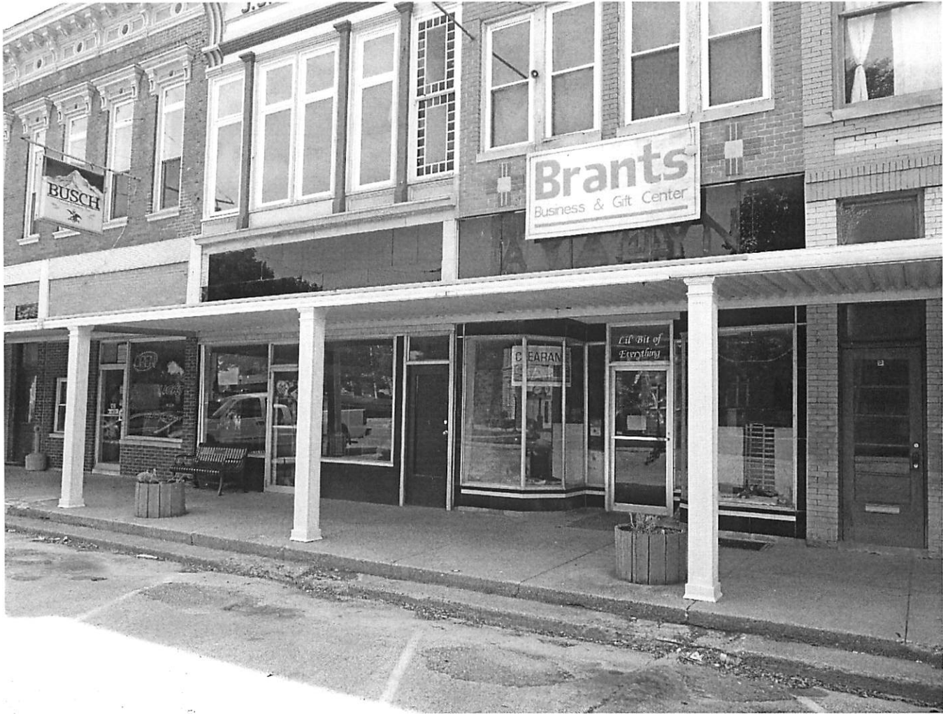
Figure 5. Adjacent mid-1930s structural glass storefronts on Madison Street, Pittsfield, Illinois.
