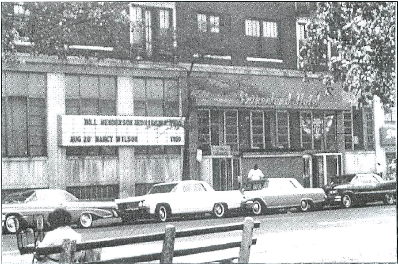
Entrance to the Sutherland Lounge on west elevation during the 1960s.
