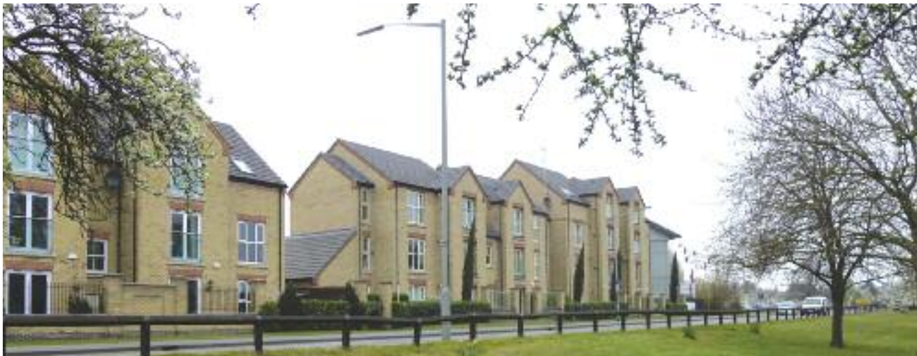
Redevelopment at Ouse Walk, Huntingdon
