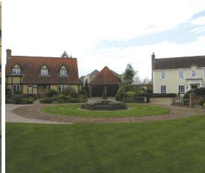
Potton Homes Showhouse complex at Mill Lane, St Neots
