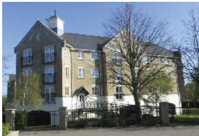
Retirement Housing, Crosshall Road
