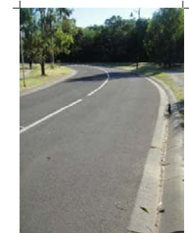
9. Bitumen Entry Road Charcoal Concrete Roll Over Kerb
