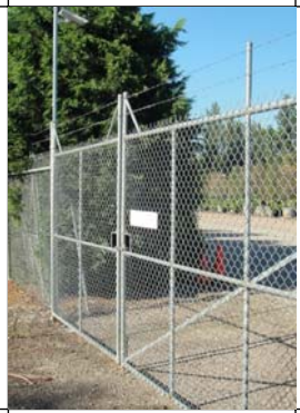
2. Kilby Tree Farm Boundary Fence/ Gate
