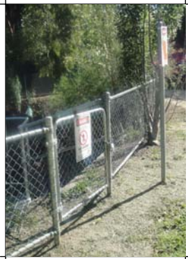
1. Melbourne Water Drain Culvert Barrier
