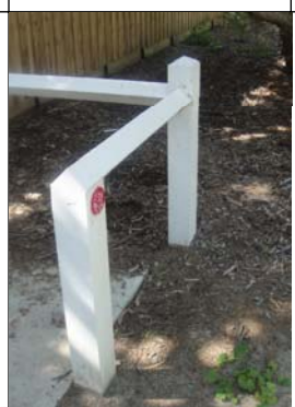
7. Painted Timber Barrier
