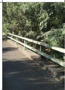
6. Glass Creek 'Bridge' Barrier
