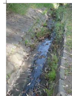
1. Old Bluestone Culvert
