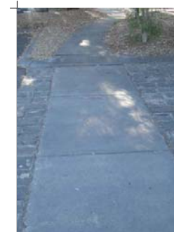
8. Carpark Bluestone Rubble Strip
