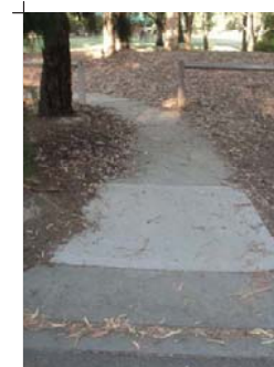
7. Charcoal Concrete Footpath
