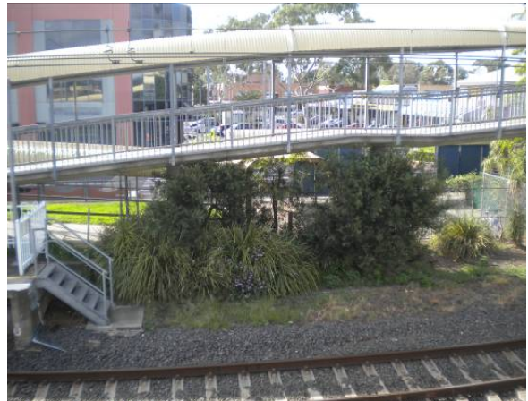
Ramp and southern end of Platform 2
