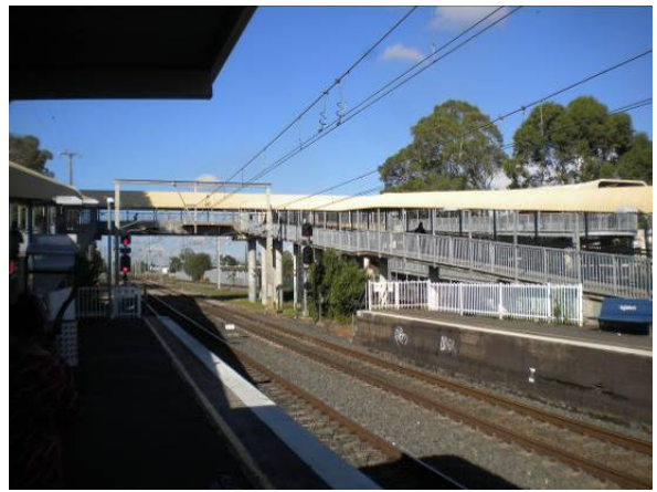
Non DDA-complaint ramp to Platform 1
