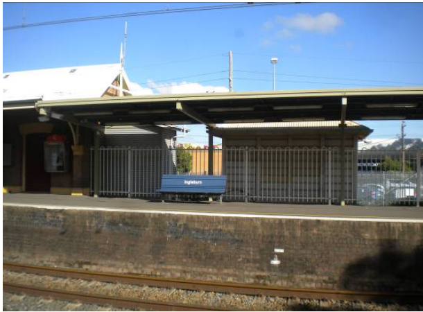
Signal box on Platform 1
