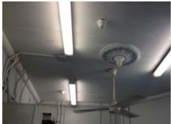
Ceiling in heritage platform building
