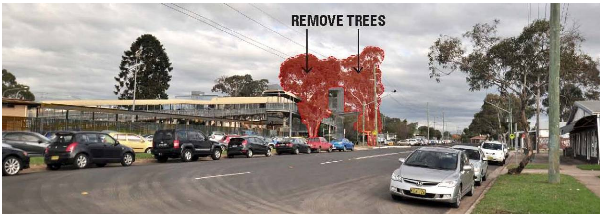
View 7A: View from Stanley Road (north of the station) indicating proposed works.
