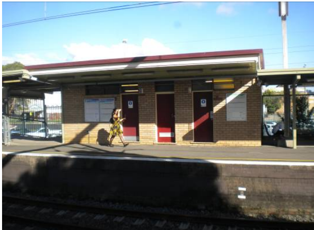
Amenities block narrows available space on Platform 1
