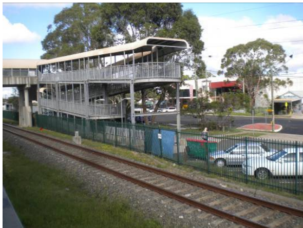
DDA-compliant ramp on Stanley Road side
