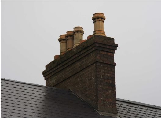
Photo 4; West View Tce.
