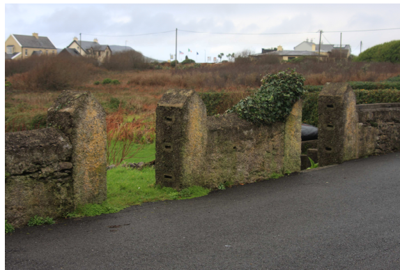
Photo 16: Boundary wall West View Terrace
