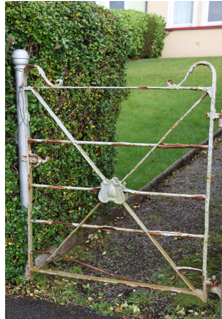
Photo 11; West View Tce.
