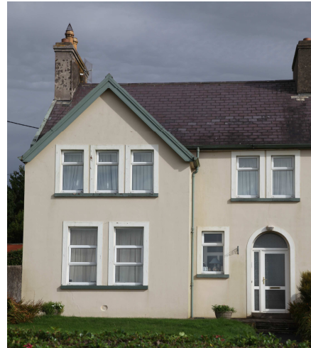
Photo 9; West View Tce.
