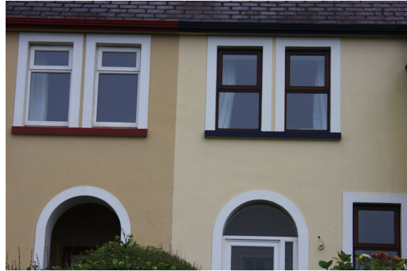
Photo 8; West View Tce.
