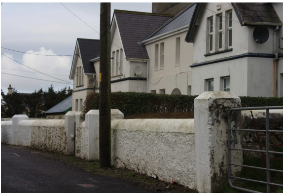
Photo 12; South View Tce. boundary wall.
