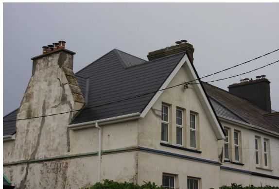
Photo 6: Existing gable end chimney stack.
