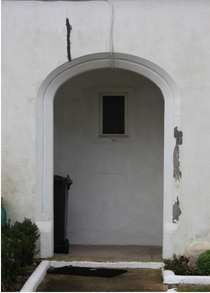
Photo 7; Entrance, South View Tce.
