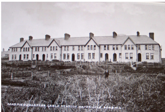
Photo 2: West View Tce. No.1-7 1880-1914
