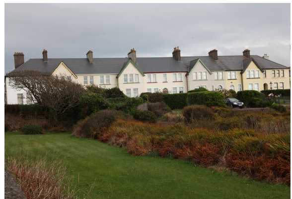
Photo 3: West View Tce., No 1-7 (2012)
