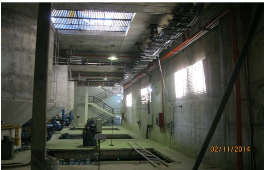
Figure 12: Powerhouse turbine floor
