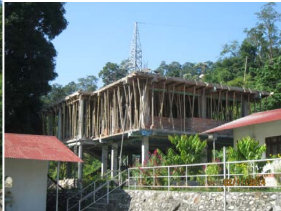
Construction of New Quarter at PH site.
