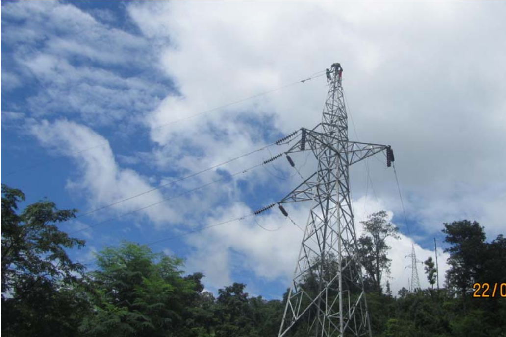
Figure 16: Transmission line progress
