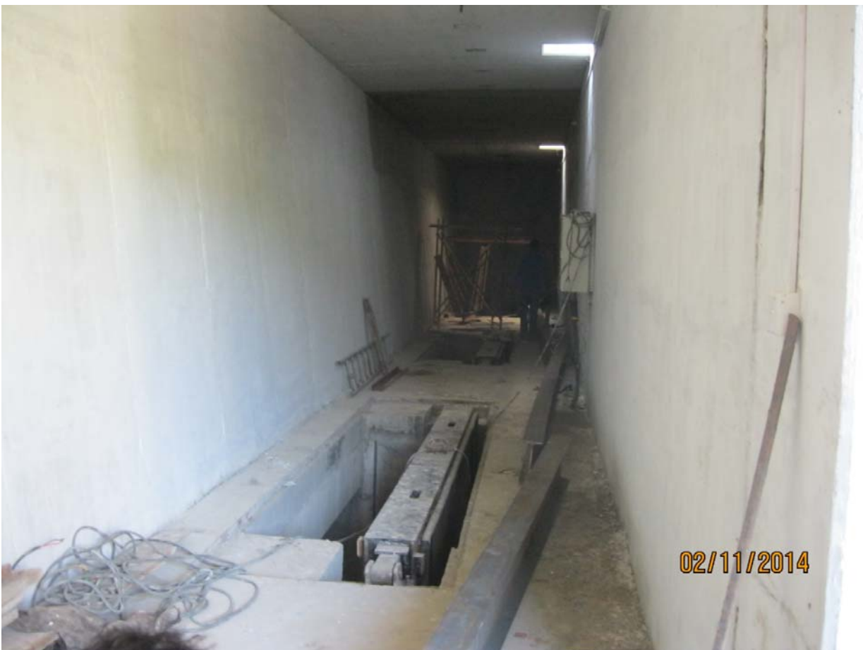
Draft tube gate area
