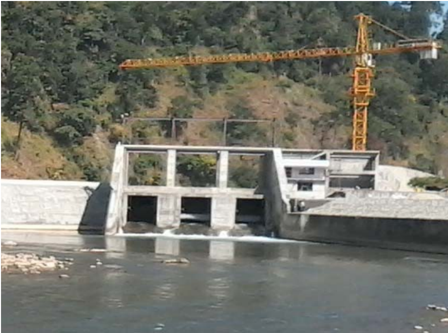
Intake from downstream
