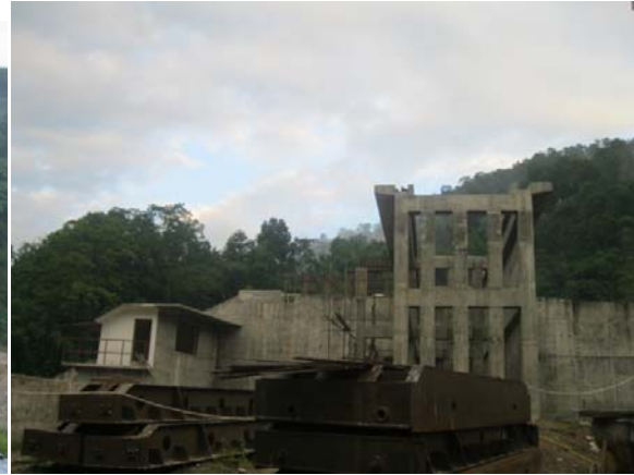
Hydraulic room and stoplog parking area
