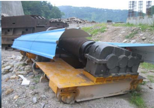
Hoisting EOT Crane on intake-undersluice delivered to site
