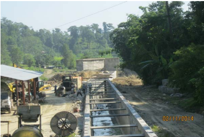
Figure 9: Tailrace extension works
