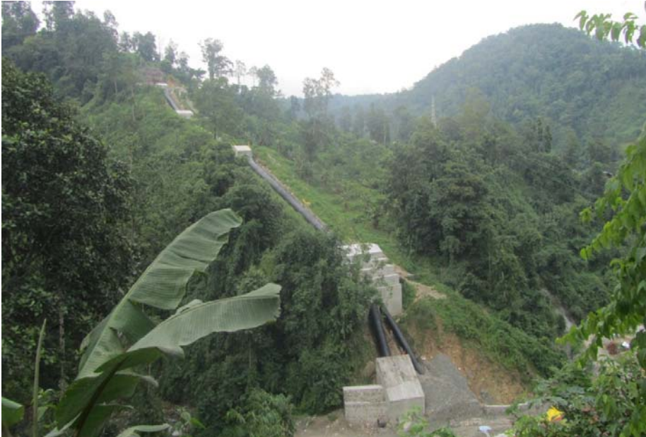
Figure 10: Penstock alignment
