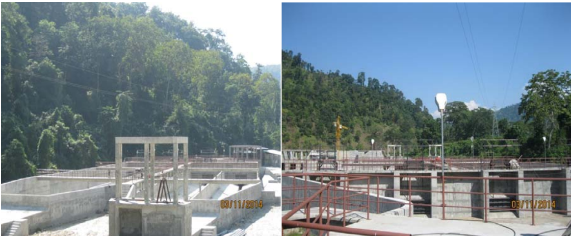
Figure 4: Settling basin inlet gate, completion of railing work of settling basin
