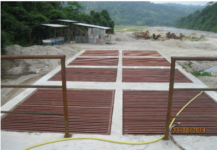
Figure 5: Grating on HRC transition top slab
