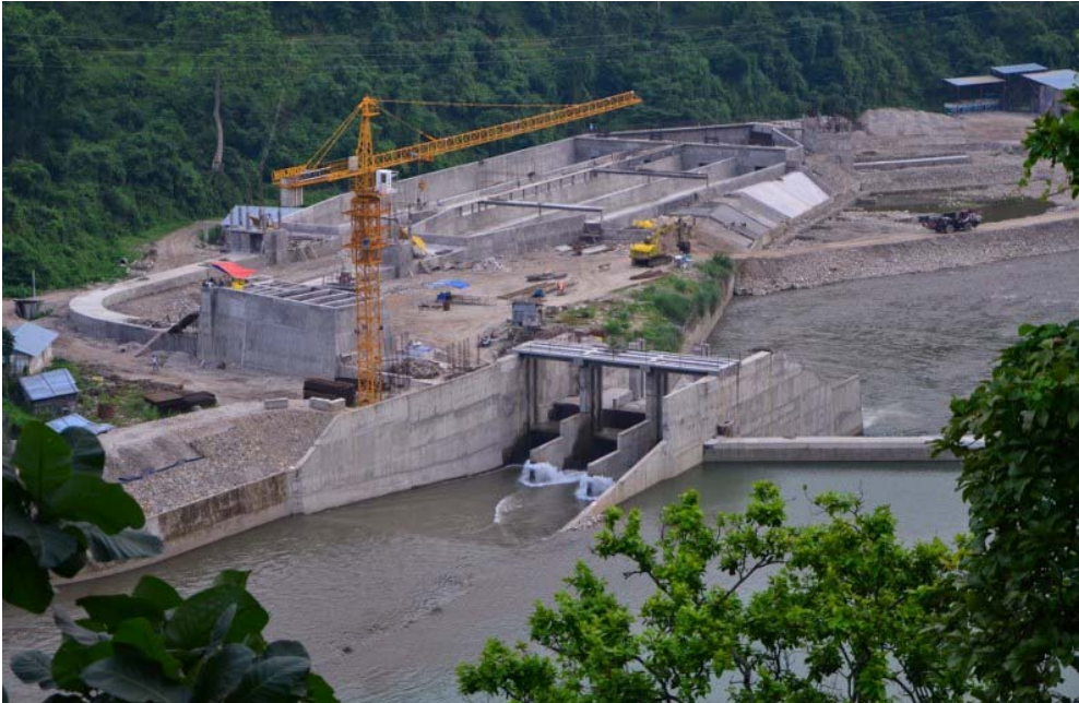
Figure 2: Upstream view of weir, intake and settling basin
