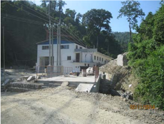
Construction of bridge and cable duct/front view
