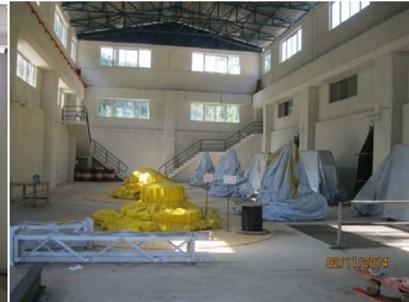
After EM installation and whitewash painting
