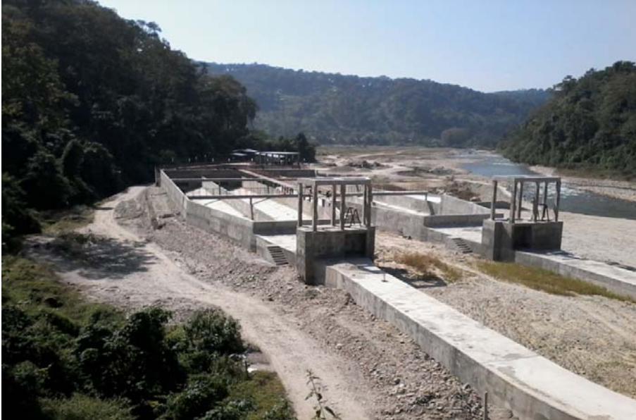
Settling basin area
