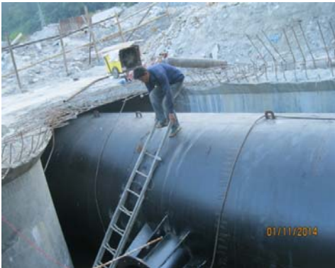
HRC access during pipe work.
