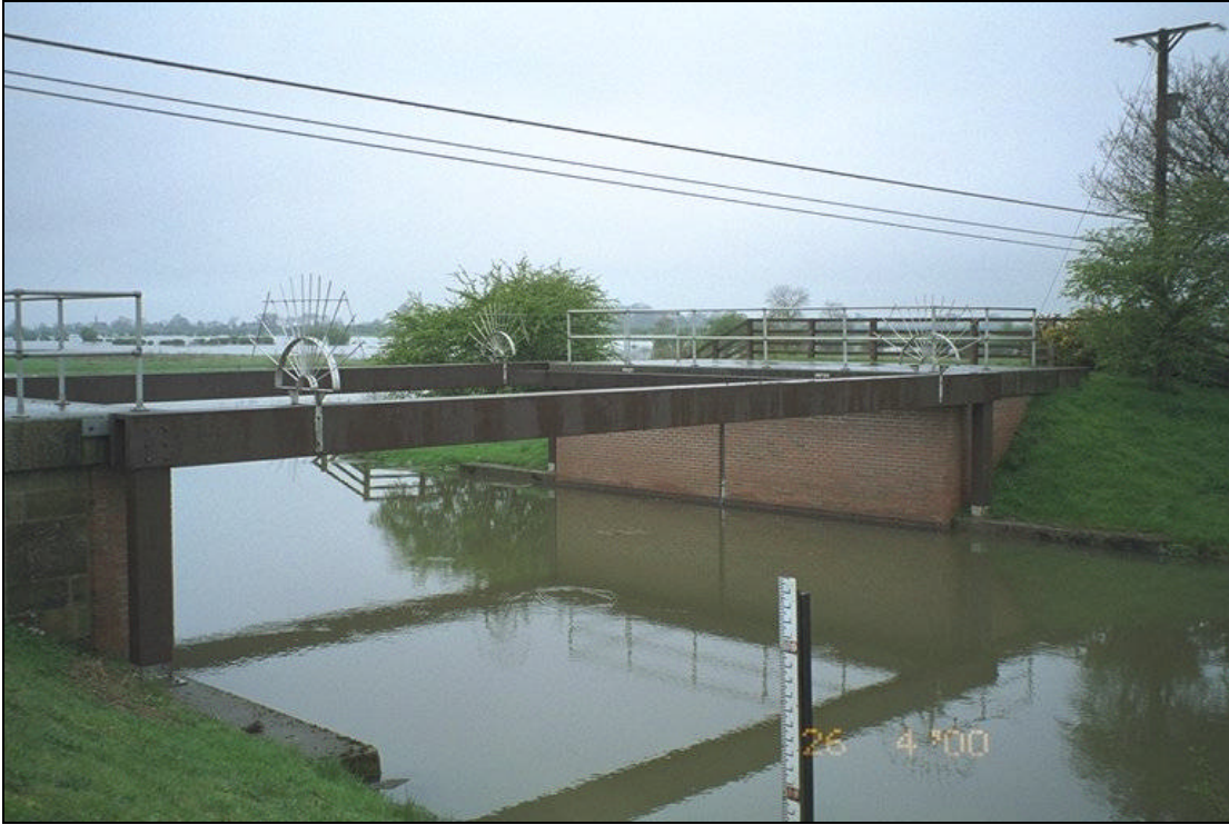
Photograph 3 River Derwent gauging facility at the position of the original bridge.
