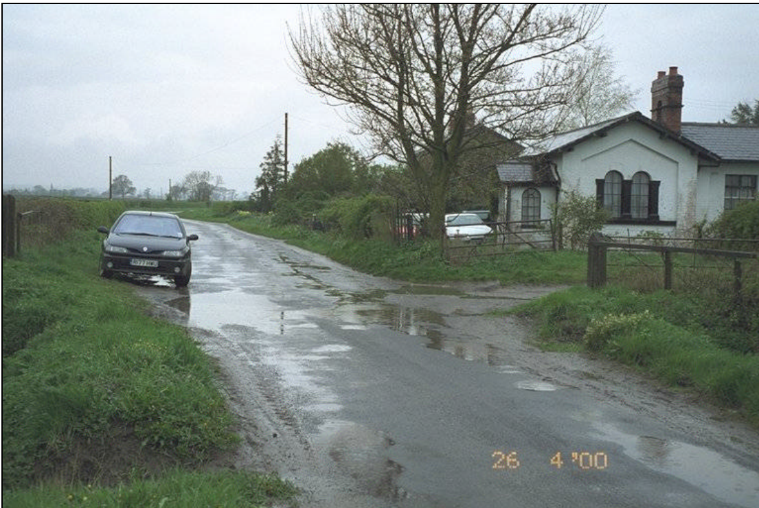
Photograph 4 Position of the original level crossing on Low Marishes Road.
