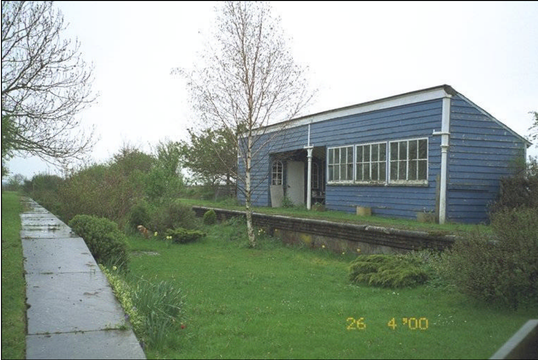
Photograph 5 Original platform forms south of Marishes Rd / Thornton Lane.
