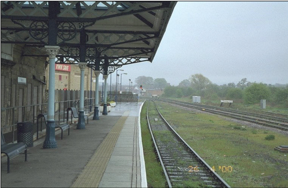
Photograph 1 Malton Station viewed towards Rillington and Scarborough.
