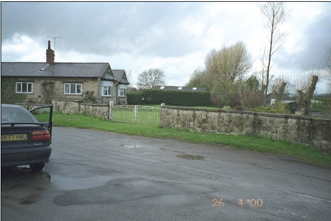
Photograph 6 Original route from the original Upper Carr Lane level crossing viewed north-west towards the A169.
